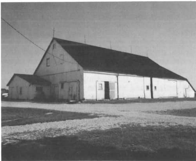
Mike Roessner owns this gable-roofed barn at 3910 Wabash Road, Fort Recovery. Five lightning rods stand across the ridge of the roof. Many of Mercer County's barns have the three openings in the gable end wall, but not many have square windows in the double doors, as this barn does. In the past, the barn was used for milking cows, and for the hay storage. Today, the barn is used for steers and horses.
