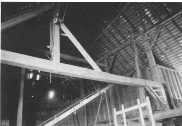
This interior view of the Evers barn shows the granary, as well as the mow for storing hay and straw for the cattle below. One can also see the framing of the barn; note the mortise in the cross beam which holds the tenon of the vertical post above it.
