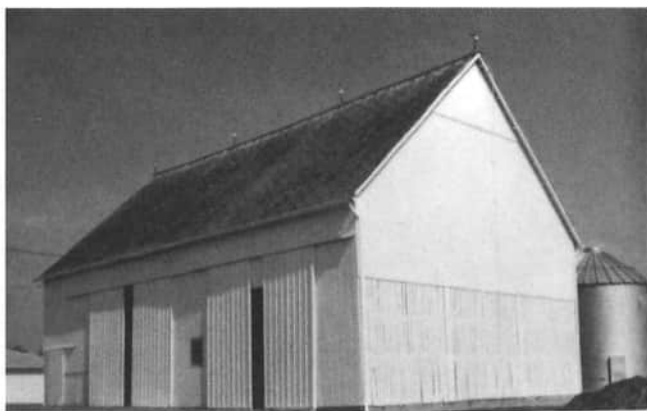
Basil E. Davis' barn, 5009 Shelley Road, Rockford, was originally a self supporting hip-roof, until the tornado in 1948, at which time the present roof structure was built. In 1990, new doors and track were added. The barn was built in 1919 by William Squires.
