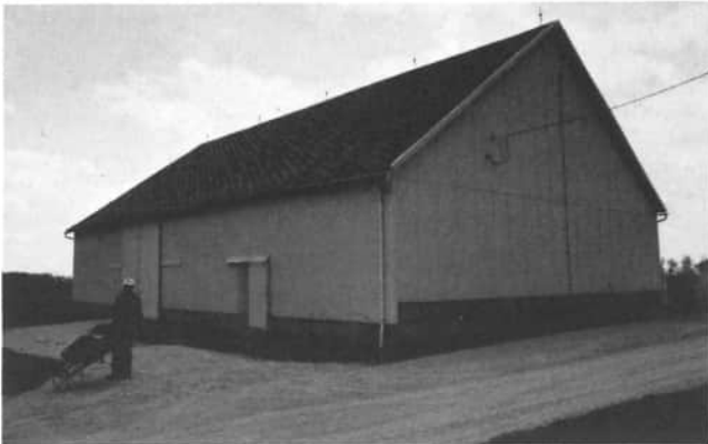
John Ronnebaum, 3881 Chickasaw Road, Celina, owns this barn. His Grandfather John B. Ronnebaum bought the farm from his great-grandfather Henry Ronnebaum on June 4, 1883. The main frame of the barn was ax-hewn logs, into 10 x 10 posts to needed length. The posts set on 6 to 8 inch thick and around 12 inch wide and 16 inch long limestone rock. It had a wood shingled roof and a wood siding. It also had a wooden floor except in the horse and cow stables. It also had a hay fork and track to pull and lift hay into the hay mow. The barn was built by neighbors and one was considered a straw boss, around 1890. The barn has since been remodeled with a new cement foundation and flooring, siding and a new roof in the 1970's.
