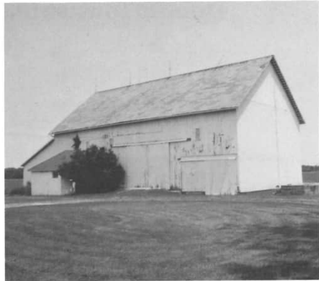
Beatrice Pifer's barn, 663 Strable Road, Rockford, was built nearly 150 years ago. In the past, the barn was used for livestock. The lightning rods still stand across the ridge of the gable roof. A slight rise goes up to the double doors. Three louvered vents allow for ventilation in the barn. Note the barn stands without a lot of other buildings next to it, in this rural setting.
