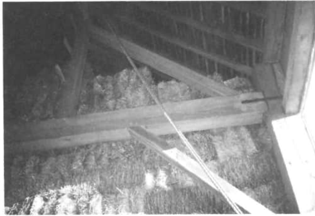
This interior view of the Thieman barn shows the huge beams supporting the rafters. The mow is full, almost to the rafters.
