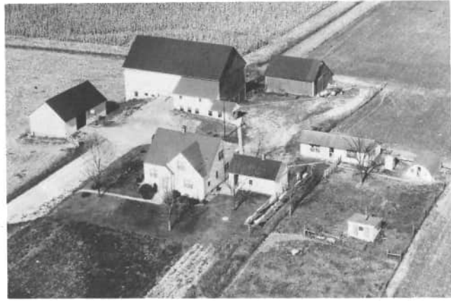
This 1956 aerial view of Ivo J. Goettemoeller's farm, 3821 Lange Road, Saint Henry, shows how the barn looked in the past. The bank goes up to the main floor of the barn. The barn was probably built in the early 1900's. The barn housed dairy head, stored feed and bedding, and stored the wagon, etc., in the center.
