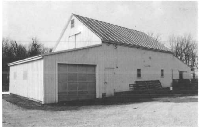
Rick Bruns' barn, 3231 Chickasaw Road, Celina, was built in 1900 by a Mr. Solmon. The barn was used for livestock and for grain and hay. Then, in 1966, the barn was torn down and rebuilt. It still has the same standing seam roof as it did when the structure was built in 1900. Today, the barn is still used for livestock and hay.
