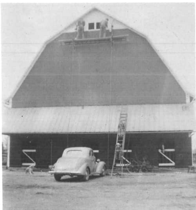
Albert and Louis Pohlman are painting the barn; the white triangle is a decoration. The stable doors are open; the horse is looking out the east side of the south end. The kick-door with the Z bracing kept the horses in. The porch roof, or pent roof, protects the stable doors. The 1936 plymouth coupe belonged to Louis Pohlman.
