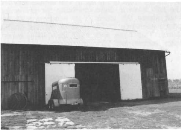
Sue Counterman's barn, 8279 Hoenie Road, Celina, was built in the 1890's. This barn originally sat on Morrow Road, on the north side of this farm. The barn was moved by Jackson Movers to its present location, around 1950, by the heirs of Jim Morrow. This barn still has the wooden hay track in the top of the barn. Four lightning rods stand across the ridge of the gable roof. The old wagon wheel remind one of the days when the horse did the pulling. Next to the wheel is a horse trailer to remind one of these days when the horse is being pulled. In the past the big old barn was used for livestock and feed storage. Today, this barn is used for horses and machinery storage.
