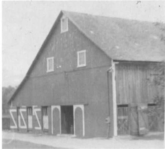
This 1950 photograph shows Robert Guggenbiller's barn before the white siding was added, and the doors and windows were covered. Note the three windows in the gable end, as well as the three braced stable doors, and the two sliding doors trimmed with white arches, at 2577 Fox Road. In the past, the barn has been used for a loafing barn, and horse stalls, with a threshing floor. Corn fodder was on top. The milkhouse and parlor were added in 1960.
