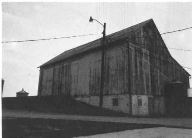
Tom and Barb Schlarman, 3164 State Route 119, Saint Henry, have this big bank barn. The barn is used to house cows and to store straw and hay. One can enter the bottom floor through the door on the side, while the tractor can still drive the big equipment up the bank to the main floor.
