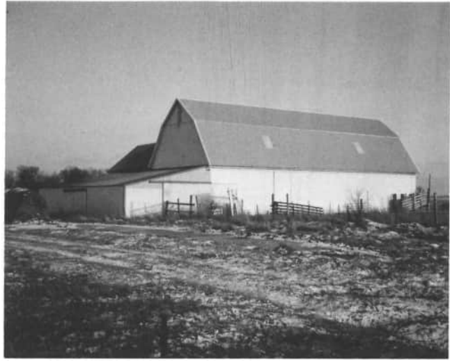
The Krieg barn is located on the Gary Krieg farm, 5618 Indiana Ohio Stateline Road, Fort Recovery, Ohio, and was built by Gary's Grandfather John Krieg, around 1912. (See the next photograph for the barn raising.) This view was taken from the north (front view); the dimensions are 72 feet by 115 feet. The lean-to on the southeast side was added in 1952; the lean-to on the north side (shown) was built in 1980.
