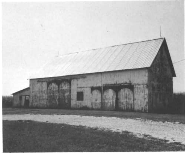
Jeff and Carol Hayes' barn, 9615 State Route 118, Rockford, write that their barn was built in 1838, by Frank Buck. The farm was bought from the government. In the past, the barn was used for cattle, pigs, horses, and hay. The gable roofed barn has a lightning rod at both ends of the roof. Dark arches highlight the sliding doors. The stable doors, topped with rectangular windows, can be seen on the end wall.
