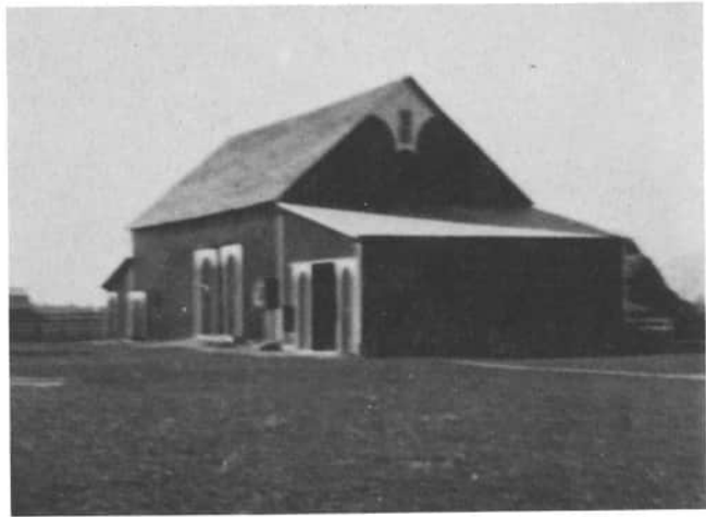
This 1942 photograph shows the same barn, belonging to Stanley and Marie Samples, after a lean-to and corn crib were added to the barn. Note the partial white arches in the gable peak. This design is usually found in northwestern Mercer County, but not often in southern Mercer County. This barn was taken down, and replaced with a pole barn, for machinery storage.
