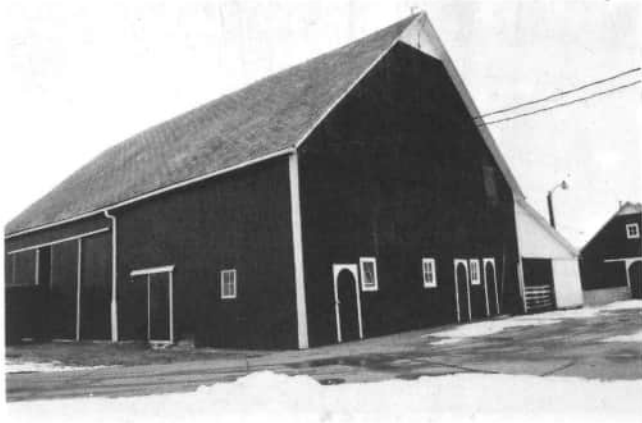
Lavern Wolters' barn stands at 5405 Siegrist-Jutte Road, Coldwater. This red barn, with the gable roof, has the white trim, with arches on the smaller doors on the end wall, capped with a white triangle at the gable peak. Note the entry to the mow; not many barns have this protected entryway. The barn was built between 1890 and 1895 by Ed Goecke. Work horses and dairy cows lived in this barn, with the grain and hay stored in the barn. Today, the barn is used for dairy cows and hay storage.
