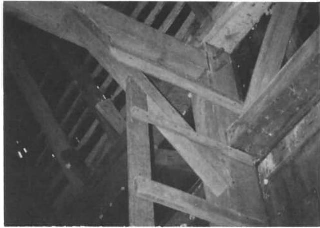
An interior view of Tim Kennedy's barn shows the wooden pins pinning the post and beam which support the roof. (Doris Glass photograph)
