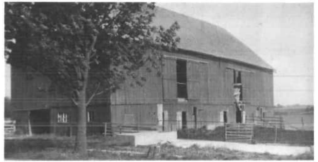
This large bank barn used to set on the Dale Dippold farm, 3804 Cassella/Montezuma Road, Celina. The Frank Heyne family owned the farm and they no longer had use for the barn; the barn also needed a lot of work done to it. So they decided to tear it down in the mid 1950's. On this photograph, the bank is on the other side of the barn. On this side, the two pairs of double doors at the level of the threshing floor can be seen. They could use these double doors to open and throw hay down to the cattle; they could also open these double doors at the time of threshing.
