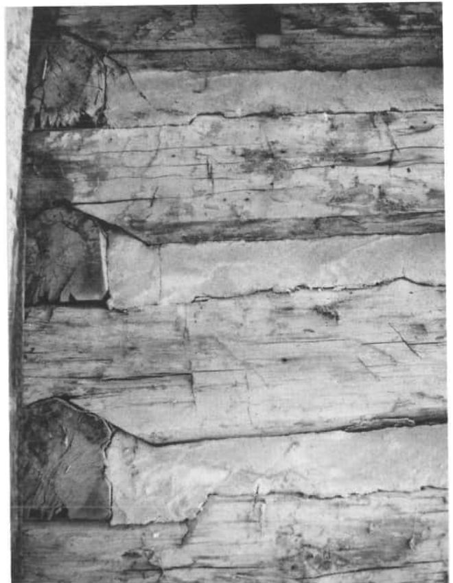
A closer view of the steeple notching of the corners.
