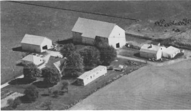
This photograph was taken of the Jerry Clune farm in 1974. Note the bank leading up to the double doors; a covered-bridge connects the bank to the barn. One of the double doors has a small door in it; this small door within the larger door is called a Guichet.
