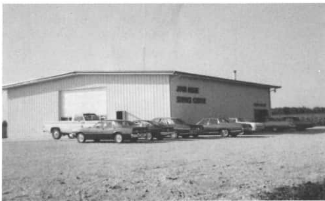
Service Center, 10991 St. Rt. 49, Willshire, Ohio
