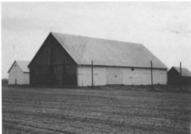
Victor Bergman, 325 North Walnut, Celina, owns this barn which is located on Clune-Stucke Road, St. Rosa. The barn was built in 1890 by an Ording. The barn was used for livestock; now it is used for storing machinery. Note the slope of the roof, in contrast with the width and length of the barn. Note that the dark wood on the barn is the original wood, that has never been painted; only the East, North, and upper part of the South sides are the original wood, without paint.
