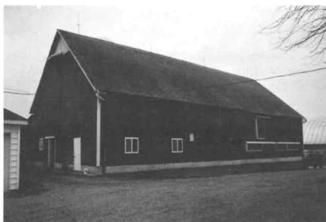
Walter Broering's barn is located at 981 Huwer Road, St. Henry. The red barn is trimmed in white. Beneath the white triangle in the gable end wall, note the hay hood over the mow entry. In the past, the barn was used for housing and milking cows, for storing hay and straw. Today, the barn is used for housing dry cows, smaller calves, and hay and straw.
