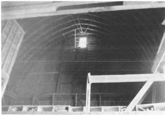
An interior view of Calvin Houts' barn shows the vast space available which the gothic or rainbow-roof made possible.
