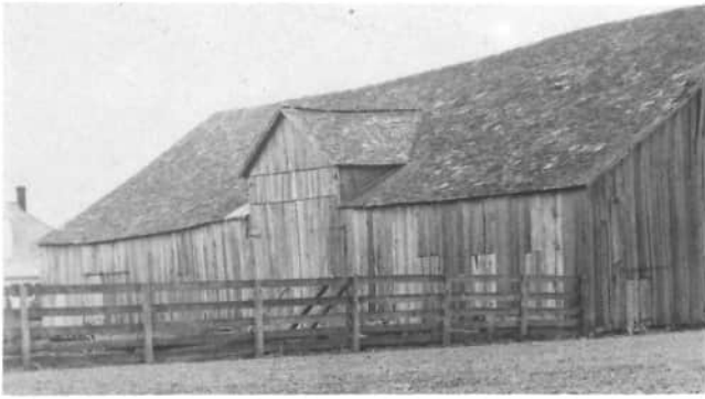
This is the old barn which stood at 3688 St. Johns Road, and was torn down in 1953, for George Bruns to build the new barn.
