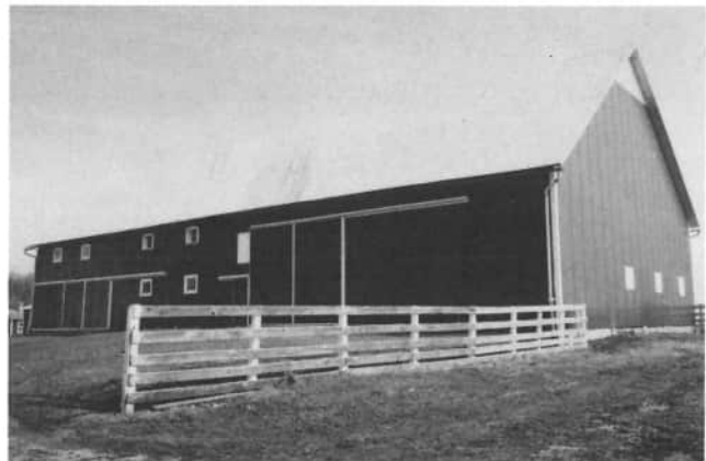
Ben and John Luttmer's barn, 7450 Minster-Fort Recovery Road, Maria Stein, was built in 1886 by Joseph Beckman and his brother. In the past, the barn also housed horses, but now houses cattle, oats, hay and straw. In the Labor Day 1947 tornado, the doors were blown off the barn, and the roof was partially torn off.
