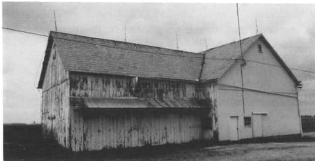
Joe Muhlenkamp owns the barn, on its original site, at 218 Elm Road, Fort Recovery. He bought the farm from his father, Ott Muhlenkamp, in December 1988. The barn is built in a T shape, with a pent roof on the side for protection over the four doors for horses.
