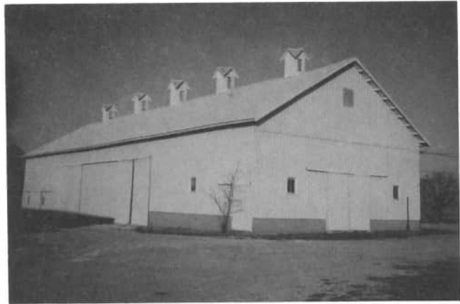
This barn on the Lee Winkler Farm on Wabash Road was built around the late 1870's, as primarily a haybarn with louvered wall ventilators and its five vented roof cupolas. It was quite large for that time, measuring 110 feet by 40 feet. It originally had a full plank floor and the big doors were hinged and swung out. There were several box stalls for horses and overhead grain bins. As farming practices changed over the barn's long history, it has been updated as needed with new siding, cement floor and foundation, sliding doors, and a rolled standing seam tin roof over the original wood shingles. Several years ago it was covered with steel siding and roof to better maintain it for current farm use. Martin Winkler homesteaded in Blackcreek Township about 1837 and the farm has remained in the family since that time. The big brick house which was built in the 1880's still is in use today, and is considered the Homeplace by the entire Winkler family. For information on this barn, the person to contact would be Lee Winkler's son, Nicholas Winkler, 795 Winkler Road, Willshire, Ohio. (Sondra Samples Photograph)
