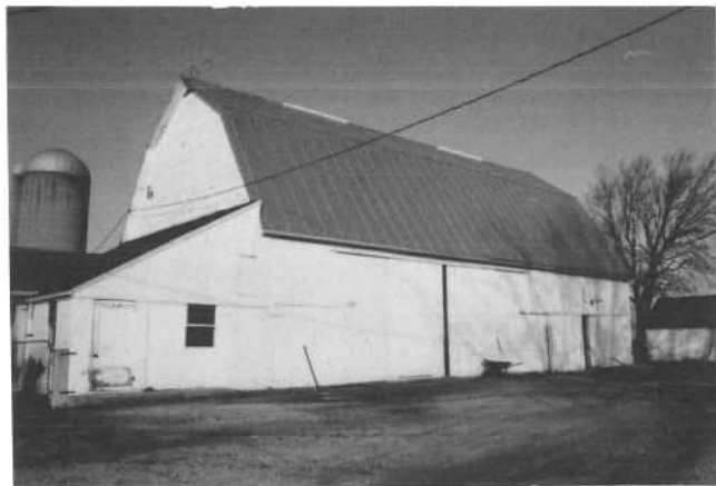
The early morning sun is casting shadows across Paul and Margie Dirksen's barn, 6791 Mercer-Darke County Line Road, Maria Stein. The original barn burned down when they were threshing wheat in the summer time. The barn today was built in 1934 by Bill and Ado Tumbusch. They worked for a dollar a day, plus their meals. Dirksens use their barn as a dairy barn. The gambrel roof allows for more space in the mow.
