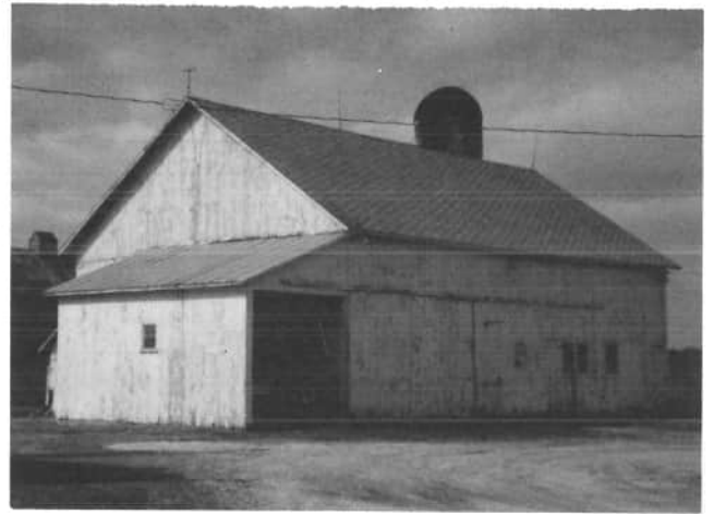
Ole K. Sites' barn, 9582 U.S. 127, Celina has three lightning rods standing across the ridge of the gable roof. The barn was built in 1892, possibly by the Brookharts. This barn has had a shed roofed addition added to the left end wall. A few windows are across the front. Behind the barn is standing a silo, and a corn crib, with a "top knot" on the roof. (Dave Slusser Photograph)
