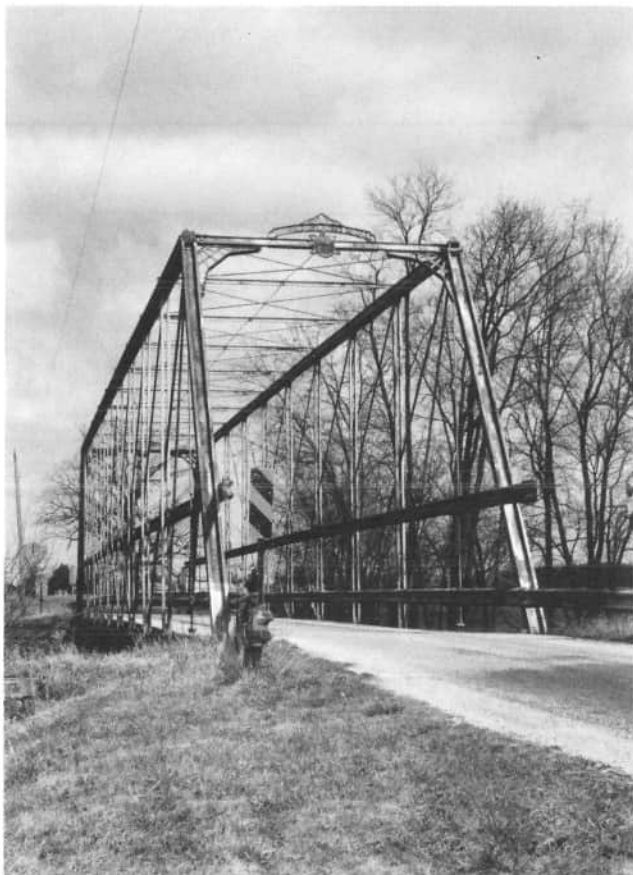
The Gallman Road Bridge over the St. Marys River is a Double Intersection Pratt (Whipple) Truss built in 1887 by the Columbia Bridge Works of Dayton, Ohio. This bridge was constructed of wrought iron and is 153 feet long. The decorative portal is meant to resemble spider webs. This bridge is currently a selected bridge on the Historical Register.
