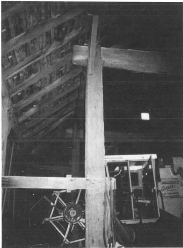
This interior view of the Jerry Clune barn, shows the cross beams as they extend through the mortises of the vertical posts, just inside the double doors. The tenons extending through the mortises and then being rounded off, is a rare sight in Mercer County barns. Barnologists (those who study barns) compare this type framing with Dutch framing of barns. Of course, another barnologist will state that this is a German bank barn!
