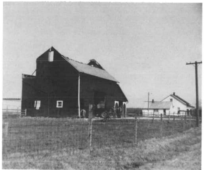
This is the 1948 view of the previous barn, belonging to Basil E. Davis. The March 19, 1948 storm took its toll on the barn. Even though the white arched barn doors are still on the front at the side, the roof is gone.
