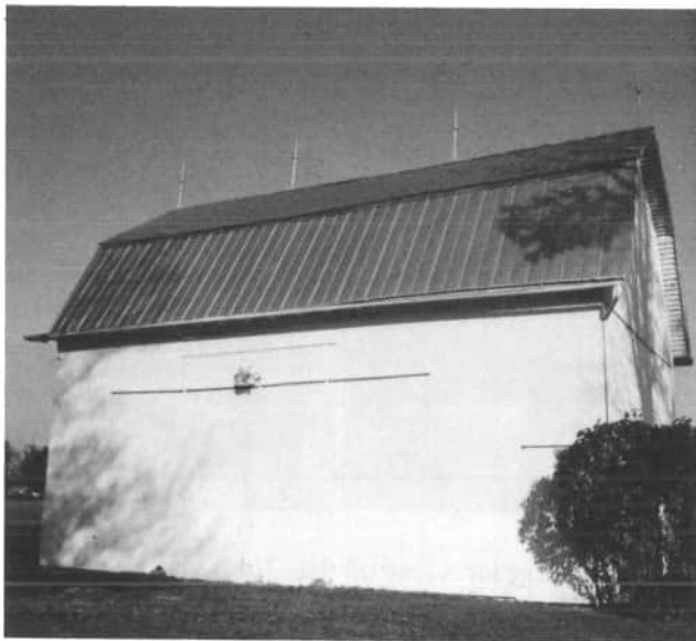
Paul and Lela Siebert, 8560 State Route 197, Celina, own this barn. Four lightning rods stand across the ridge of the gambrel roof. The barn stands much as it did when it was built.
