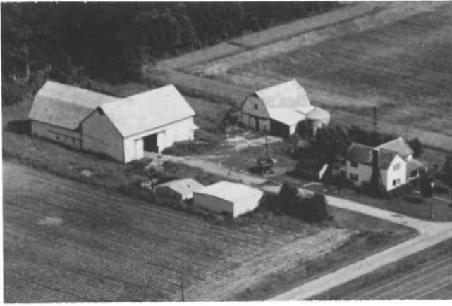
This aerial view shows the William Frit-zinger's barn and other buildings at 8710 Linn Road, Celina. The main barn has a gable roof, with a barn built behind it, with a gambrel roof. In the past, the barn was used for cattle, horses and grain. Today, the barn is used for storage.
