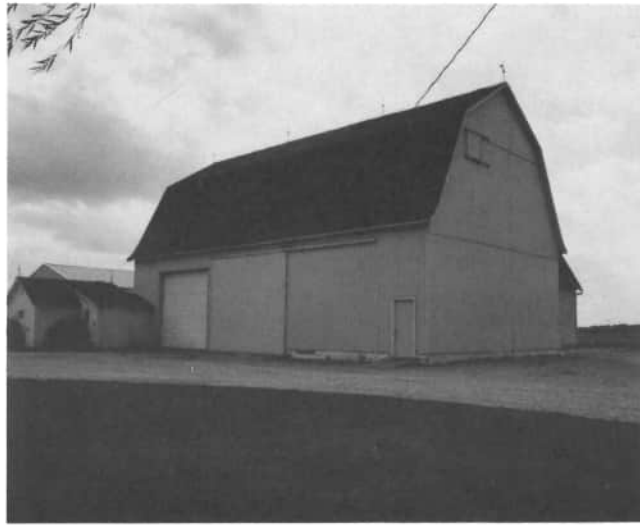
David Hileman, 9471 Erastus-Durbin Road, Rockford, owns this barn with the gambrel roof. D. R. Smalley built this barn, and this barn has been used for raising cows. Today, the barn is used for storage of grain and equipment.
