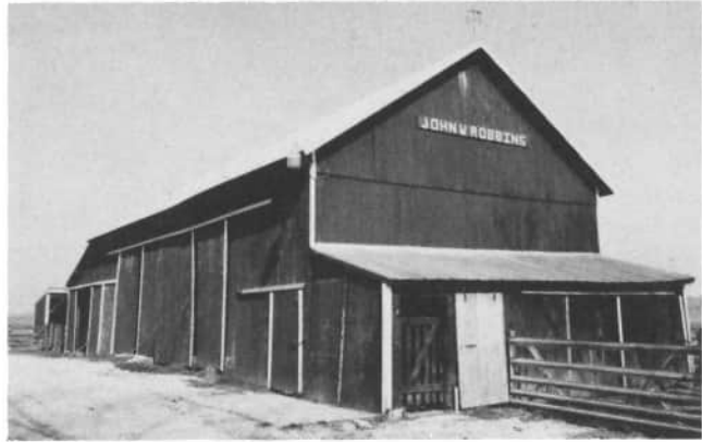
John W. and Naomi Robbins' barn, 8149 Wabash Road, Celina, was built from hewn timbers, and pinned with wooden pegs, 1895-1900; the rafters are round native timber. The owner's name, John W. Robbins, is printed across the end of the barn. (Putting the owner's name on the barn is almost a lost art in Mercer County.) This barn has been used for livestock, machinery and hay storage. In 1992 this barn presently houses Belgian Draft horses, which are used for work, pleasure and profit.
