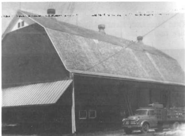
The finished barn is 44 feet wide, 84 feet long, and is 40 feet from the foundation to the peak of the barn. Four lightning rods and three ventilators are on top of the barn. Mr. and Mrs. Albert Pohlman, (son of Mr. and Mrs. Henry Pohlman) got the farm in 1942, at 1809 St. Rt. 716, Maria Stein. This farm has been in the Pohlman family since 1837; they have the sheepskin deed, signed by President Martin Van Buren.
