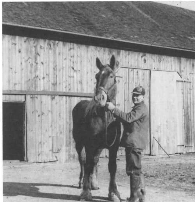
Wilmer Hoenie and his horse Dick are standing in front of the Hoenie barn at 8404 Hoenie Road. The lightning rods can be seen on the gable roof ridge. The double doors are braced open, and they opened on a hinge.
