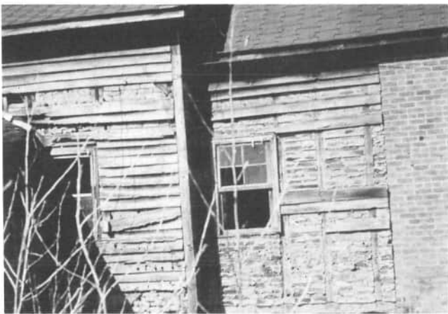
Figure 2. Half-timber construction in an abandoned house in Western Ohio
