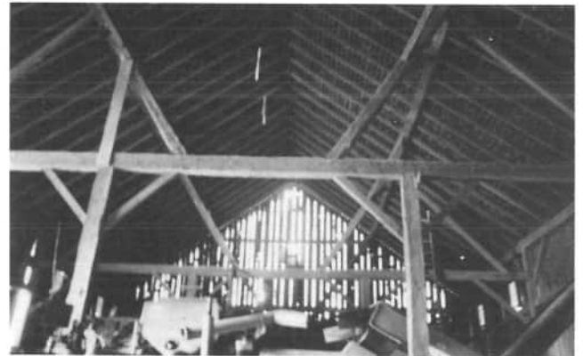
This interior view of Edson Pierstorff's barn, not only shows the symmetry of the framing, but also identifies a unique type of framing. Note above the main cross beams, that the inclined posts are supporting the purlin. Most Mercer County barns have vertical posts supporting the purlin, beneath the rafters. This type framing suggests that the builder had knowledge of shipbuilding from the east coast, because they used these inclined support posts for the ship they were building. At the end of the barn, the sunlight outlines the vertical boards.
