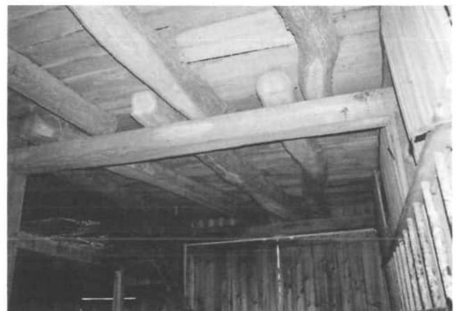
The hayloft beams still have their bark on the sides, in Don Wellman's barn.
