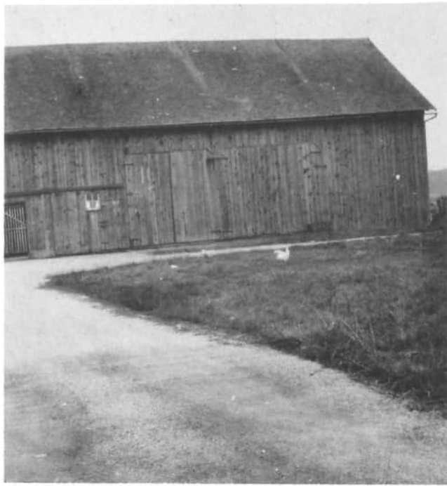
George and Norma Hoenie's barn, 8404 Hoenie Road, Celina, was built in the 1870's by their Uncle Charlie Frahm. This barn was built out of native timber and the beams were hewed out by hand and pinned together. The original doors swung open on hinges.
