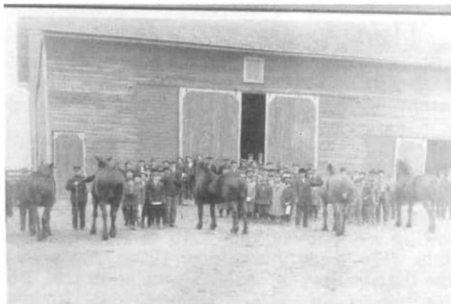
This view of the completed Baker barn, shows the window above the double doors; which are trimmed in white, with the white triangles at the top corners of the doors. This barn was 104 feet long on the west side. One year, five little colts were raised and later broke and used for farming. "Our treasured trees," 47 acres, were donated in 1991 to the Ohio Department of Natural Resources, to be known in the future as the "Baker Woods Preserve."
