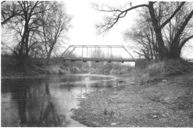
The Wabash Road Bridge over the Wabash River is a full Pratt Truss built in 1886 by the Buckeye Bridge Company of Cleveland, Ohio. This style was prevalent during this period. Surviving bridges are still frequent.
