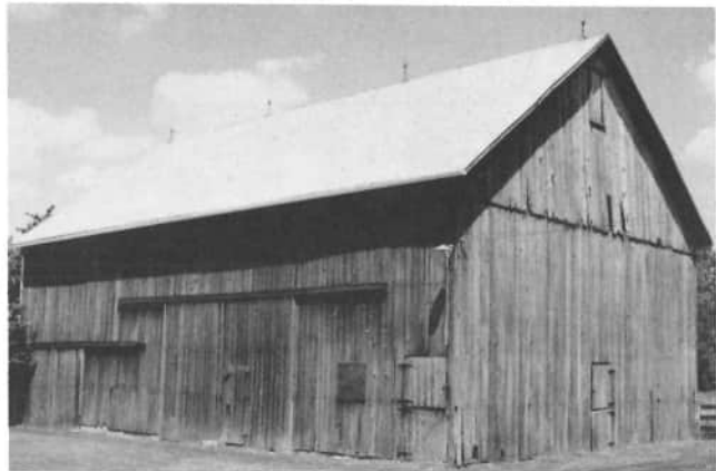
This fine barn, weathered to a fine patina, stands at 5056 McMillan Road. The barn was built for John and Margaret Boley at the turn of the century; the barn is 60 feet by 40 feet; the cross beams are sawed and are forty feet long. Almost a century old, the barn still stands straight and tall. Four lightning rods stand across the ridge of the gable roof. John and Margaret Boley's Granddaughter Connie (Boley) Johnson now owns the place.
