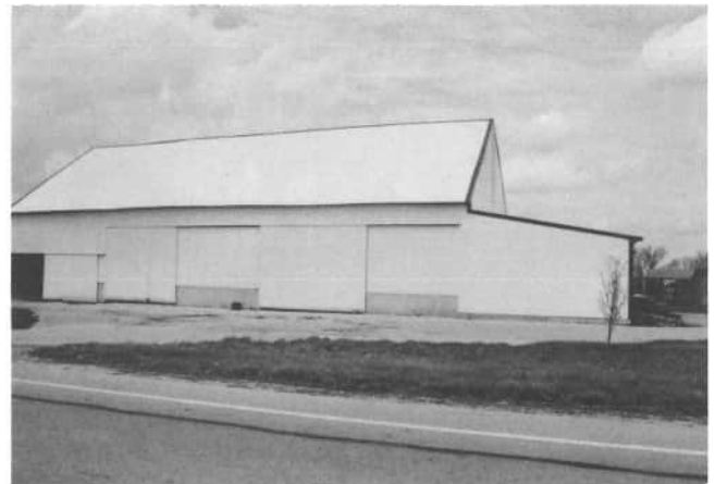
Larry Dwenger's barn, 3215 State Route 29, Celina, was built in the early 1900's. The barn was used for dairy in the past, and is used for steers and hogs today. They redid the barn in 1988. The gable roofed barn has an addition to the right. If one looks closely, one can see the small service door, cut into the large sliding door; the smaller door within a larger door is known as "le petit guichet."
