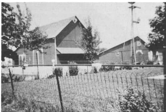
This barn originally stood on the northeast corner of the intersection of Hone-Weir and Burrville road; in 1938 it was purchased from the Kendall's by Ezra and Nellie Laffin and moved to its present location at 7780 Burrville Road. Note the pent roof on the end; the barn is also trimmed with white arches. A white diamond decorates the gable end; this is an unusual design in barn decorations of gable ends.
