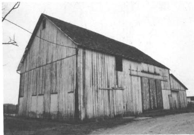
This barn was built in 1907, with hewn logs and wooden pegs, by Jacob Huwer. Horses were located on the east side of the barn; the horse stable doors can still be seen on the end wall. Milk cows were housed on the west side of the barn. Straw and hay were stored in the barn. This place was in the Huwer family until it was bought by Bernard and Mary M. Siefring on June 15, 1970. The barn will possibly be torn down in the near future, because of its poor condition. At present, the barn is used for hogs and for storing straw. The barn stands on the west side of the road, and belongs to Bernard Siefring, 5130 Burkettsville-St. Henry Road.
