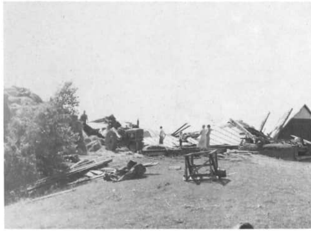
Lloyd Schwieterman's barn, 6804 Depweg Road, after the July 19, 1952 storm.
