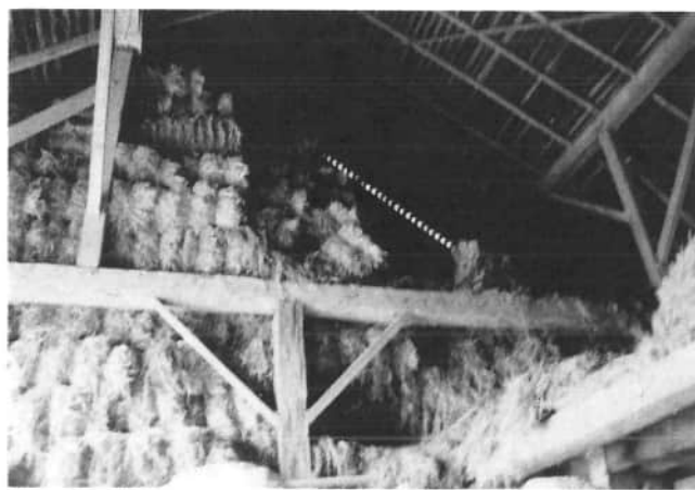
An interior view of Victor J. Homan's barn shows the framing and the hand hewn beams, as well as the vast space of the mow, at 3411 Philothea Road.
