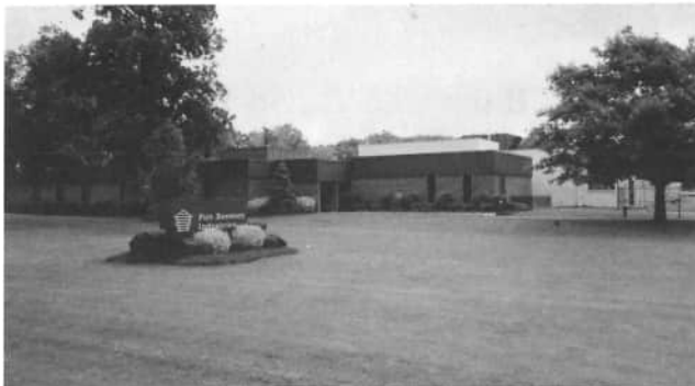
Ft. Recovery Industries, Inc. Hardware Plant
