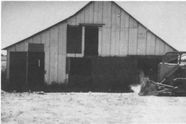
This barn was used for milk cows, and they raised hogs in it; it also stored hay and straw. This barn was at the place of Dave and Bernice Sheets, 10938 Neptune-Mendon Road, Mendon. The barn was getting in bad shape so their son tore it down with his bulldozer in 1978. Now they have a pole barn.
