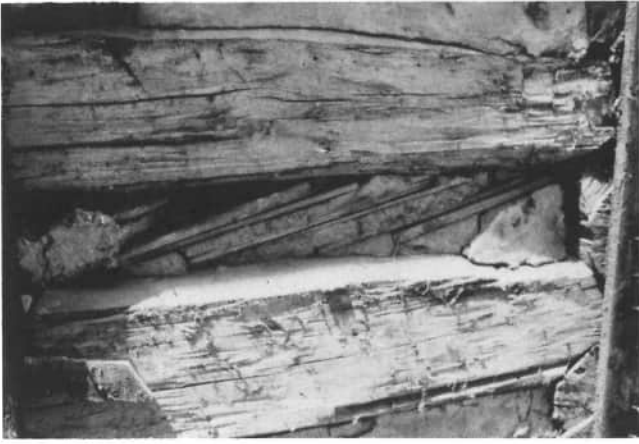
A closer view of the chinking between the logs.
