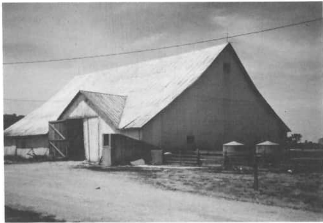
William C. Granger built this barn in 1912. The barn was used for hay storage and shelter for horses, cows and sheep. This long-sloped roof makes for an unusual entrance with its gabled roof. Herbert Siefring, 5058 Burkettsville-St. Henry Road, Coldwater, owns this barn, which is located on Karch Road. Today, this unique barn is used for storage for straw.
