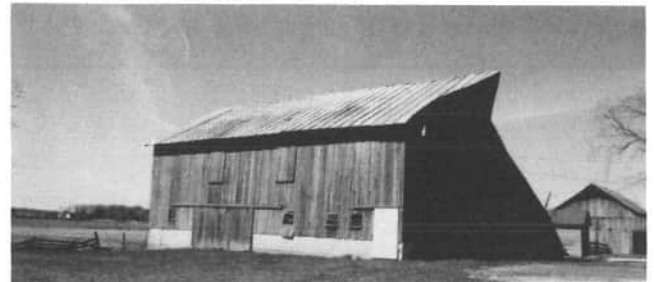
Miletus Newcomb built this barn at 6991 Howick Road, before the Civil War. The barn was used for horses, dairy and hay. Having a rich texture of weathered barn siding, the barn has a unique triangular hay hood, extending from the gable end. Today the barn is used for hay and storage, and is owned by Bonnie and Miletus Miesse, 6560 Howick Road, Celina.
