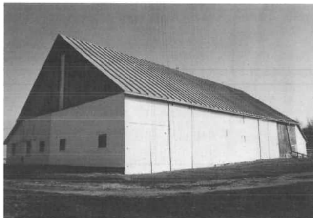
The Cyril Everman family is the fourth generation of the Everman family to live at this place, 2251 State Route 716, Maria Stein. The barn has all hand hewn beams, and was most likely built by the Everman family. The barn has been used to house livestock and for feed storage. Notice the width of the barn in contrast to the length, and notice the low slope of the roof, which is quite similar to barns built over a century ago in Marion Township.
