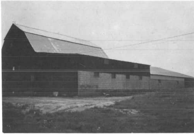
Walter Kramer's barn, 866 Watkins Road, Fort Recovery, was built in 1929. Note the steep pitch of the gambrel roof, which allows for more space in the mow. Additions have been made to this red barn. Dairy cows were in the barn, 1945-1954; then chickens, (layers), and now the barn is used for storage. The original barn at this location was destroyed by lightning in 1924. A Fordson tractor was lost in the fire. Lawrence Painter was living at this place at that time.
