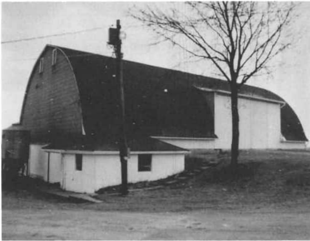
Lloyd Schwieterman's barn is unique in that few barns can tell the same story that this barn can tell. The top part of this barn was built in 1952, by Ray Stachler and the neighbors. (Ray Stachler is well known locally for his barn building.) The bank leads up to the main double doors, which fit into the roof like a large, shed roofed dormer, or looking at the slight flare at the edge of the roof, the similar flare above the doors might be called a ski-jump. This round roof, sometimes called a gothic or rainbow roof, allows more space in the mow. The bottom part of this barn was built in the 1900's. A storm, July 19, 1952, blew the top of this barn down. Lloyd Schwieterman's barn stands at 6804 Depweg Road, Celina.
