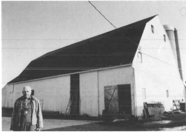
Aloys Unrast, 6015 Mercer-Darke County Line Road, New Weston, Ohio 45348, was working outside, the February 1992 day that this photograph was taken. His barn was built in 1950 by Edward Subler and has been used for livestock. Today the barn is used for dairy. Like other barns built in the 1950's, the barn roof has a gambrel roof, to allow for more storage space in the mow area.
