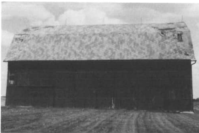
Erma Schadt's barn, 1805 Frahm Pike, Celina, may have been built around 1925. The gambrel roof has five lightning rods across the ridge. Two pairs of sliding doors are centered on the front of the barn. Two smaller stable doors are to the right of the double doors. In the past, the barn has been used for cattle, horses, machinery, some grain, and hay and straw; today the barn is used for storage.
