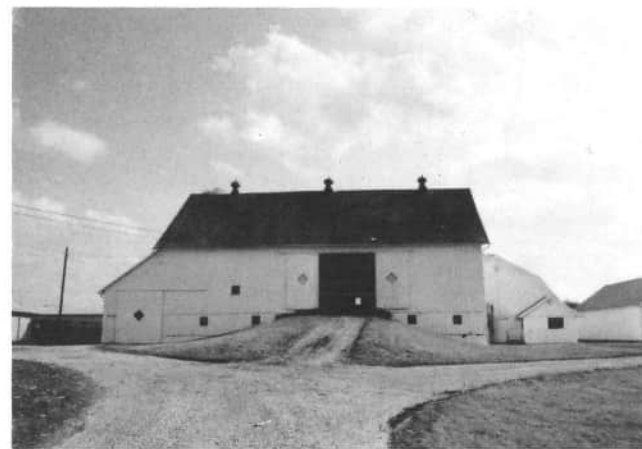
Carl Fortkamp's barn, 3818 Philothea Road, was built by Aug. Heckman before 1895. The bank leads up to the double doors with diamond windows. Three ventilators cap the ridge of the gable roof. A diamond window is also centered on the sliding door on the bottom floor. In former years, the barn has been used to house horses, cattle and hogs; today the barn is used to house reg. guernsey herd. This photograph is dated April 1992, the spring of the year in downtown Philothea.
