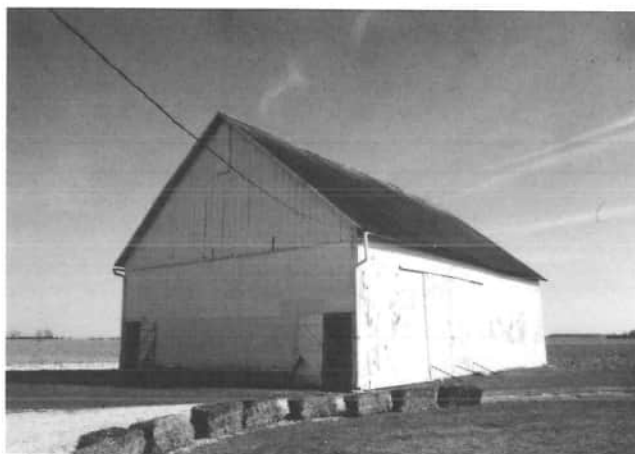
Ralph E. Fleck, 9094 State Route 197, Celina, has this English barn, also known as a three bay barn. The barn has straight, unadorned lines, with the gable roof, and was built about 1900. Traditionally, it was used for livestock and hay; today it is used for storage.
