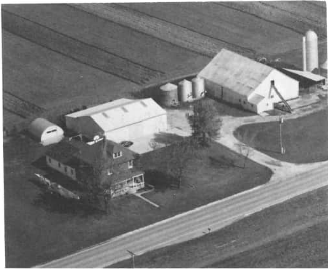
This aerial view of Martin Lefeld's farm, 3651 State Route 119, Saint Henry, shows the barn as well as the other buildings. The barn was built in the early 1900's by the Wessel family. The frame of this barn has solid hickory beams, which were made with a broad ax. The frame is wooden pinned together. The barn has always been used to house livestock, and to store hay and grain.
