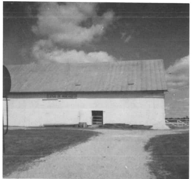
A view of the Menchhofer farm, at 1151 St. Anthony Road, after the barn had new siding and a new foundation.
