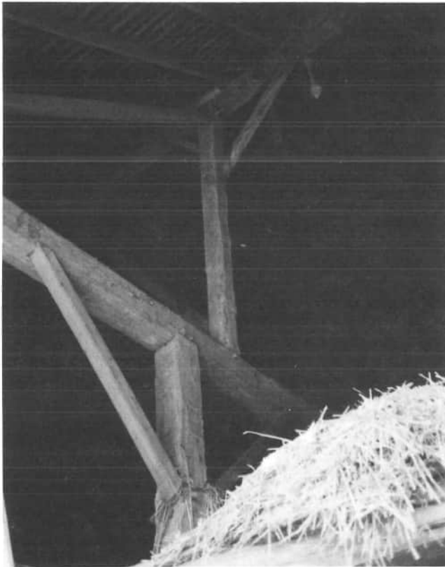
This interior view of the Hoying barn shows the hand-hewn posts and beam, which have been pinned with wooden pins.
