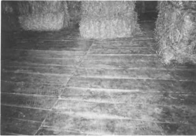
This is an interior view of the threshing floor of the Bruggeman barn.
