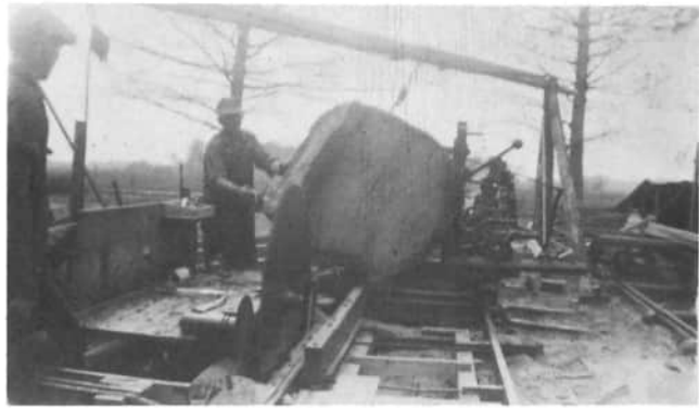
Julius Griesdorn and Al Weitzel are turning the log; the sawblade is ready to cut the slab.
