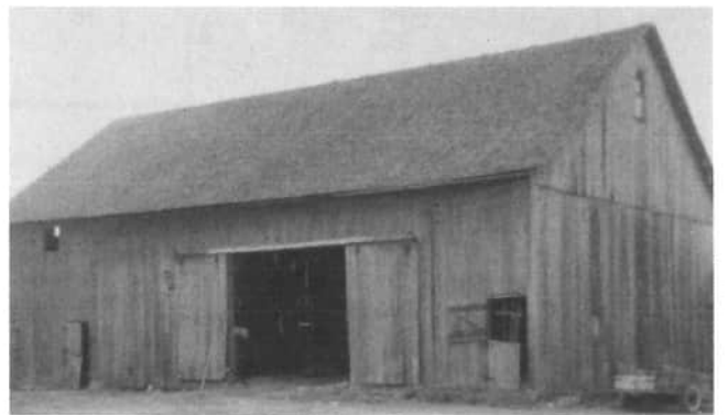
Clifford Hoffhines' barn stood the first place south of Chattanooga, on the west side of State Route 49. One can see the stable doors on the front of the barn on this photograph. One window is in the gable end wall. This barn was dismantled in 1978, and rebuilt at Bearcreek Farms, Indiana, where they took this barn and another barn together to make the gift shop.
