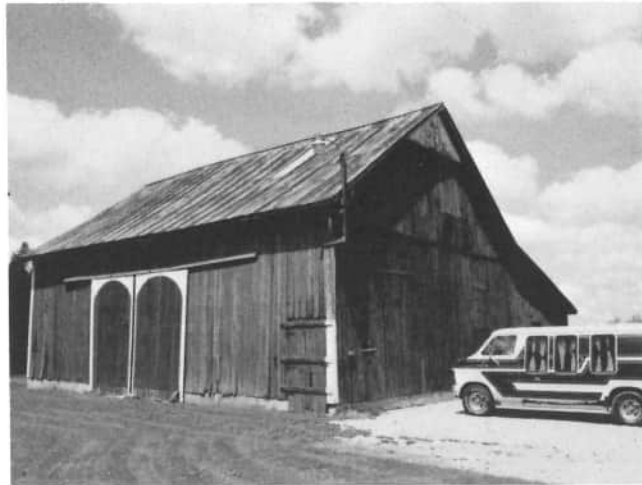
Paul Bonvillian's barn, 4105 State Route 703, Celina, was built in 1910. This barn is an English barn, with the main double doors centered on the front, and trimmed with white arches. The red barn also has a white triangle painted in the gable peak. It appears as if a new foundation has been added to the barn. Other than the addition to the back of the barn, the barn probably looks much as it did when it was built; it still has straight lines. If it were not for the night light and the van, one might not be able to date when this photograph was taken. In the past, the barn was used for animals and farm equipment; today it is used for storage.
