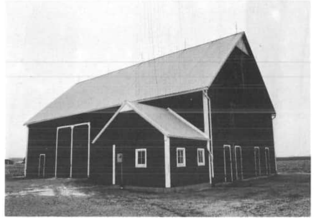
John Balster built this barn in 1934, after the old barn was struck by lightning. In the past, the barn was used for horses, cattle and feed storage; today the barn is used for feed storage and machinery. The barn is located at 5124 Carthagena Road, and belongs to Ludwig and Dolores Wuebker, 5129 Carthagena Road.
