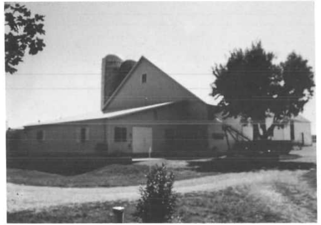
Donald B. Unrast's barn stands at 4827 State Route 119, Saint Henry. The barn is used for dairy.
