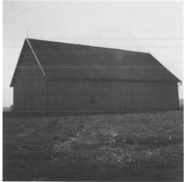
This barn was half this size at one time. It now stands in a quiet field on the east side of State Route 118, just north of the owner's home, Ivan and Dorothy Miller. This used to be Hellwarth place.
