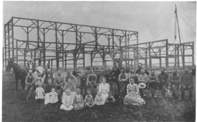
The Gin Pole is still standing, with its ropes and pulleys, after being used for leverage, in the barn raising at the John Krieg place. This photograph was taken from the East (rear) side of the building. The owner John Krieg is standing in the back row, next to the horses. The original dimensions of the barn were 36 feet by 90 feet.
