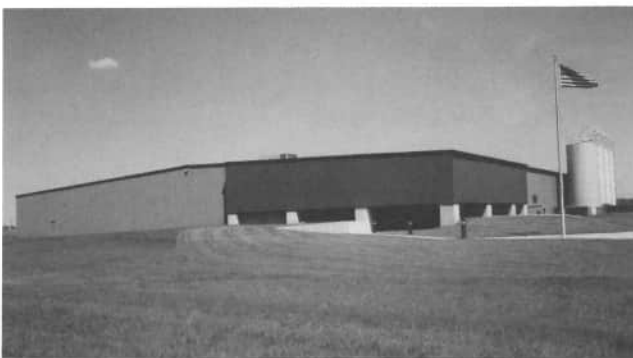
Ft. Recovery Industries, Inc. Portland Plastics Plant
