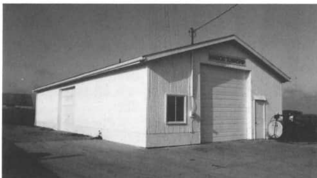
Marion Township House
