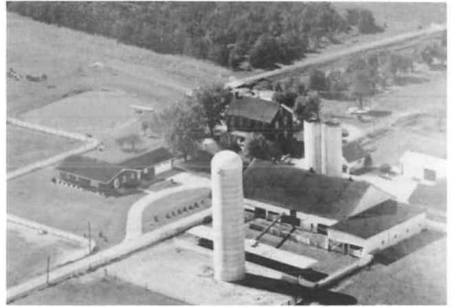
An aerial view of Dale Goettemoeller's farm, 2287 Goettemoeller Road, Maria Stein, not only shows the big barn and silos, but also the old brick home as well as the new home. Bernard Goettemoeller built this barn in 1870; with the main part of the barn being fifty-eight feet wide and ninety-six feet long. This has to be one of the bigger, and older barns of the county. This barn was added on to, in the 1890's; the flat part was added in 1950. The total length of the barn today is 130 feet! Most of the beams are hewn with an ax, and as hard as ever! Originally, the barn housed horses and cattle on the bottom, and hay, straw, wheat and oats, and feed on top. Today, the bottom is used for cattle and feed, with the top being used for hay, straw, and feed. Notice the lower slope of the roof, and the width of the barn, in comparison with the length of the barn.
