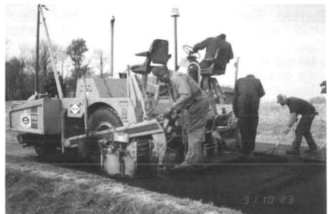
Mercer County Road Crew at work doing spot paving.
