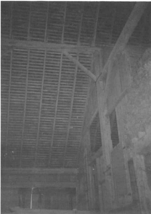
The interior view of Louis Schemmel's barn shows the granary, the mow, and the posts and beams used for the frame of the barn.
