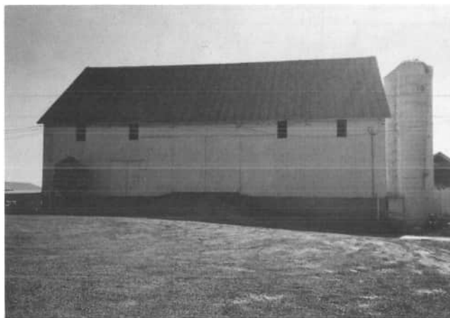
This barn is located on the Charles Schwieterman farm, located at 4339 Mercer County Road 716 A, Celina. This was the Henry Klosterman Sr. home farm; Ruben (Rub) Klosterman built the barn around 1885, out of hand hewn logs. The barn measures 46 feet wide, 84 feet long and 50 feet high. The timbers in the barn are hand hewn with pieces measuring 12" x 16" x 48' long. If one looks closely, one can see the cross beams extending through the wall, beneath the eaves. The barn has been used to house cattle, and store grain, hay and straw.
