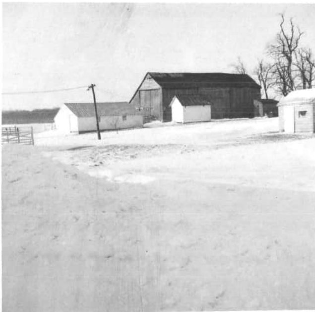
This is the old log barn, which stood on the Broering farm, when Al and Bernie Homan owned the farm. This original barn was a log barn and was built in the late eighteen hundreds when Wesley Meinerding owned the farm. Roger Schmit, a young man from Saint Henry, was hired to tear down the old barn, after the new one was finished.
