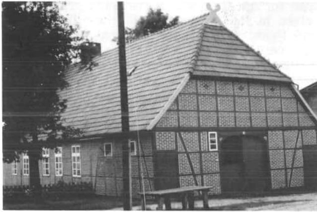
Figure 1. Lower Saxon housebarn. Note the half-timber construction and small residual smoke holes.
