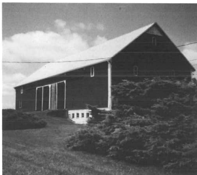
Mrs. Werner Kemper, 8739 St. Rt. 274, New Bremen, Ohio 45869, owns this barn in Marion Township. The barn was built about 110 years ago. The barn was used for hay and straw storage, and cows. Today, the barn is used for steers, hay and straw. This red barn, with white trim on the double doors, corners, and windows, has a large bank leading up to two pairs of double doors. Three windows in triangular configuration are placed beneath the white triangle in the gable end wall.
