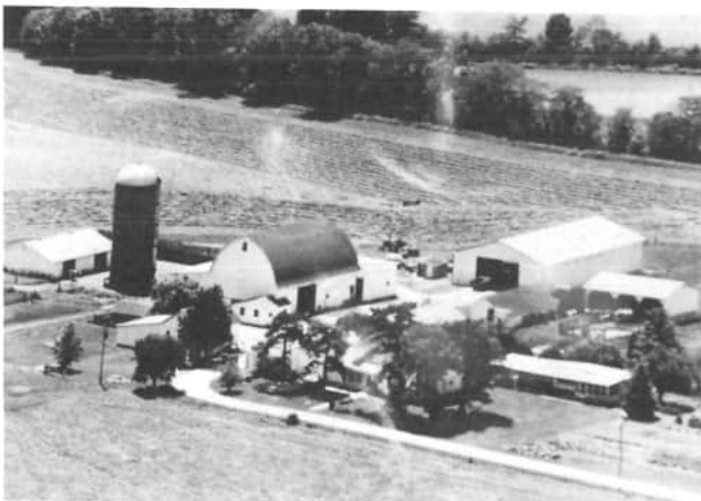
John and Don Smith and Sons, Farlane Farm, have this farm at 4370 Frahm Pike, in the family for over a hundred years, to make this a Centennial Farm. The main barn has a round roof, (also known as a rainbow roof or gothic roof), which allows for more space in the mow. Today, they use this barn for dairy, for Registered Holsteins.
