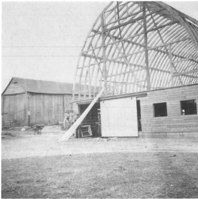
This view of the Broering barn, not only shows the structure of the roof as the barn was being built in 1956, but also shows the old barn in the background.
