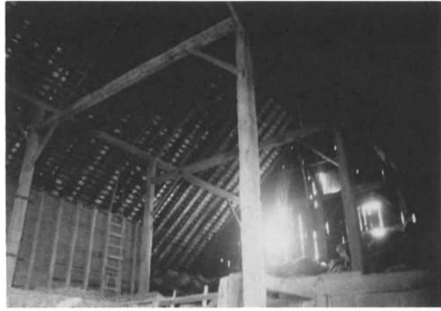
Another view of the interior of the Evers barn shows the vertical posts which support the purlin plates beneath the rafters of the roof. Anthony and Marie Evers, the former owners, now live at 1929 Cassella Montezuma Road.
