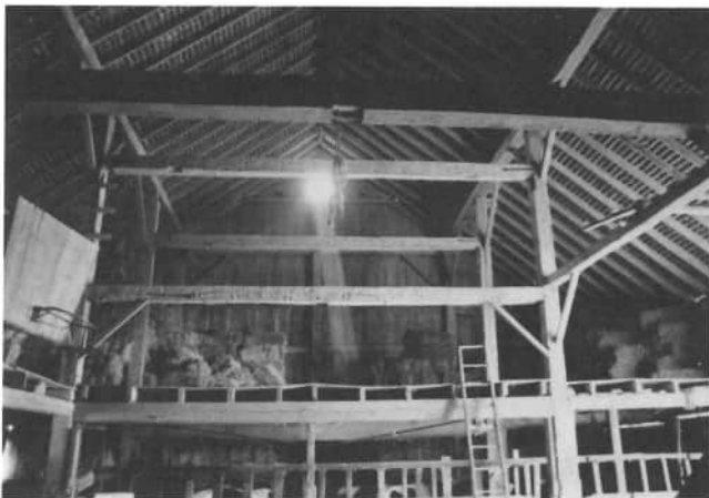
The sun shines through the window at the peak of the gable in the south end of the barn. The three horizontal, hand-hewn beams are mortised into the post which supports the purlin. The hay and straw bales are stored above in the mow, while the steers are below. The basketball board shows the younger ones play as well as work in the Bills' barn.
