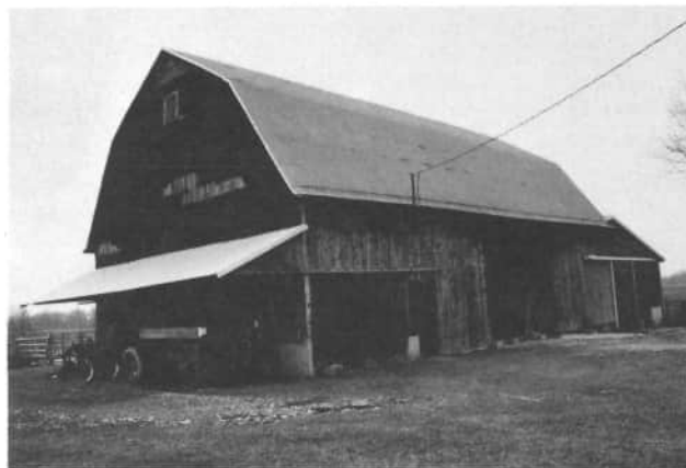
This gambrel-roofed barn has the protective pent roof on the east end of the barn. The pent roof of many Mercer County barns often is added to the east end. This barn was built in the early 1900's, and is used for livestock; today the barn belongs to Linus J. Clune, 2841 State Route 118, St. Henry.
