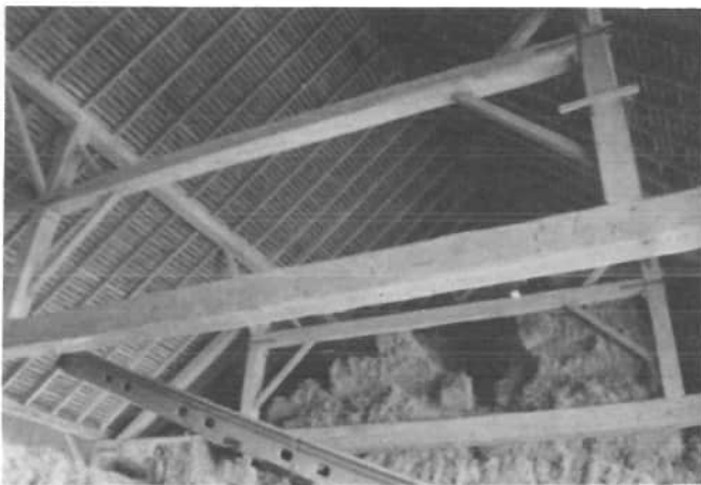
An interior view of frame of Steve Homan's barn. The two main cross beams extend through the wall, under the eaves, above the double doors.
