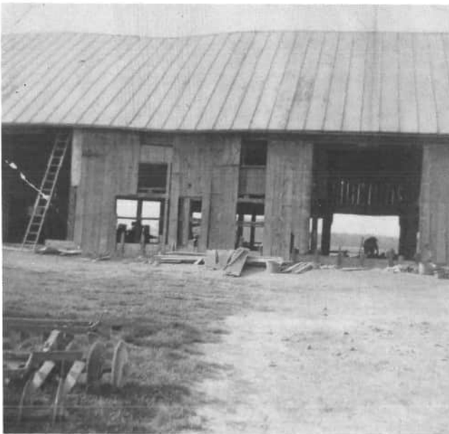
A front view of the Menchhofer barn at 1151 St. Anthony Road in May 1955. One can see the original standing seam roof, which is still being used in 1991.
