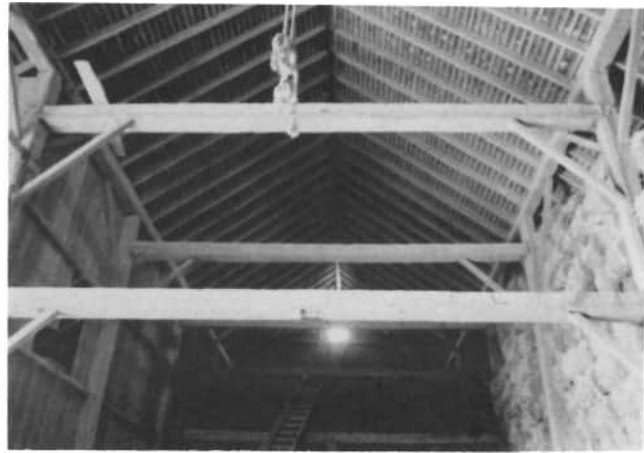
The north end of the barn shows the mow is stacked high on the right, with the grain bin standing on the left, in the Alvin Bills' barn. Note the top crossbeam is mortised into the vertical post, not at the intersection of the purlin, but just a little lower on the post. The purlin is the horizontal beam, running the length of the barn, and supporting the rafters.
