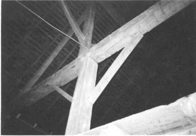
This interior view of Hart's barn, shows the old hand hewn beams, with the interlocking mortise and tenon, held together by wooden pins. These posts and beams support the purlin plate which supports the roof rafters.
