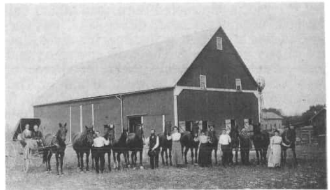
Eleanora Moeder's barn, 3799 St. Rt. 119, St. Henry, was built sometime after Eleanora was born in 1893, and before their house was built in 1909. The entire barn had a wooden floor, which included the threshing floor. The mow was packed full of straw, over the cow stable, when they were threshing. There was a cistern under the floor, near the horses. It was easy to water the young calves when the weather was bad. (Editor's note: Bernard Hummel's barn, to the east of this place, also had a cistern inside the barn.) This barn was built for Joseph and Adelheit Moeder, by a carpenter named Losekamp. In the carriage are Emma (Uhlenhake) Moeder (John's wife), and Adelheit (Haubert) Moeder, (Eleanora's Mom). Standing are John Moeder (Eleanora's brother), Joseph Moeder (Eleanora's Pop), Eleanora Moeder, Mary Moeder (her sister), Albert Moeder (her cousin and Priscilla's brother), Aloys Moeder (her brother) and Matilda Moeder (Tillie-her sister). The horses are Harry, Fan, Brauny, Dick, Nell, Sam, Bill, Mabel, Birt, Prince, and Jim. At this writing, Eleanora was 98 years old and still living on her own, in April 1991.
