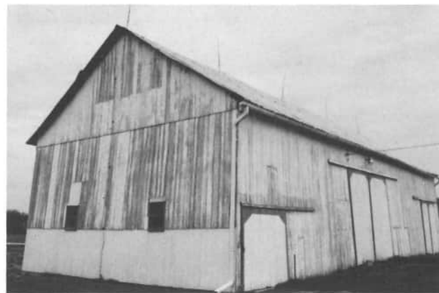
James Carter's barn, 7689 Township Line Road, Celina, was built in the 1880's and has been used for cattle, hay and straw. The timber in this barn is of hand hewn oak. The barn is 30 feet wide and seventy feet long.
