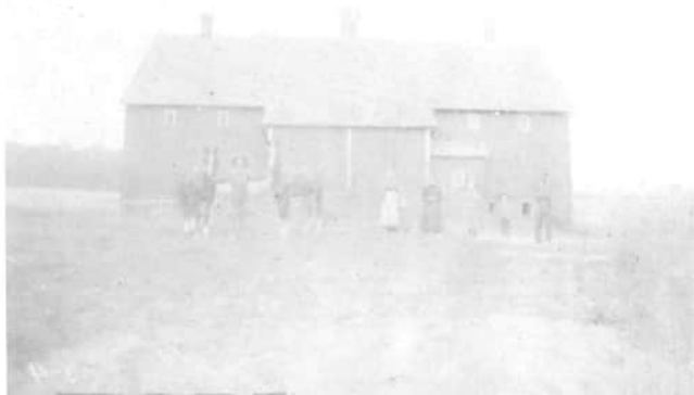
This Clune barn stood at 1414 Clune-Stucke Road, Maria Stein. The owners were Maxmilian and Maria Clune, then Herman and Christine Clune, then Clarence and Ida Clune, and today, Jerome and Patricia Clune. The family on the photograph is most likely Herman's family. The barn is 90 feet long, 48 feet wide, and 50 feet high. A previous log barn on the property was torn down and they used the logs for flooring joists for this barn; they are hand-hewn, 18 inches to two feet wide. The main beams the length of the barn have only one splice in 90 feet, with a two-foot overlap; that means 47-foot trees hewn by hand. (The three cupolas are no longer on the barn today.)
