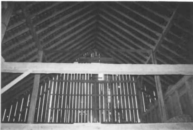
Another interior view of John Homan's barn, 97 Elm Road, shows the symmetry of the frame. The end wall's vertical boards are spaced enough to permit ventilation in the barn. The cross beams are all one piece; not spliced. Tall vertical posts support the purlin plates which run the length of the barn and support the rafters of the roof.
