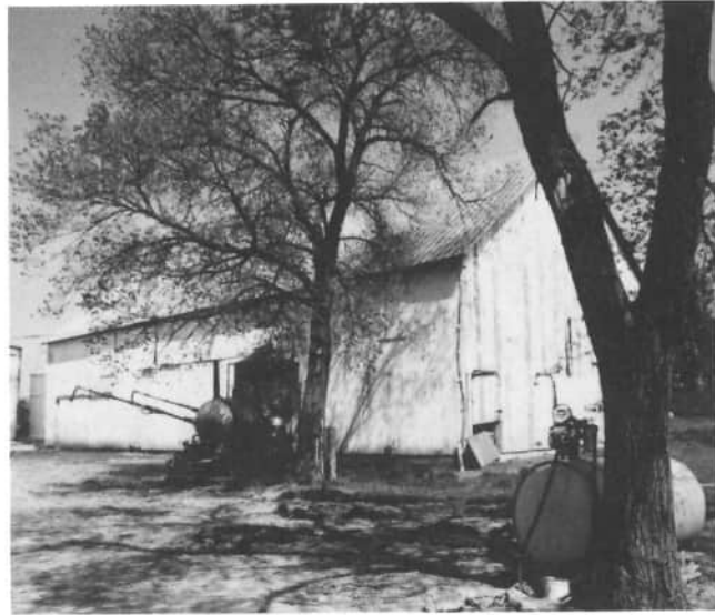
Gale Thomas, 8155 Burrville Road, owns this barn which was built around 1900 by Gale's Great-Grandfather. This barn was used to shelter the horses and cows in its early years; there also was a hay mow over the entire barn. This barn measures 96 x 38. In 1953 the barn was turned a quarter turn to set it on a new foundation, in its present east and west location. Today, the barn is used to keep hogs.
