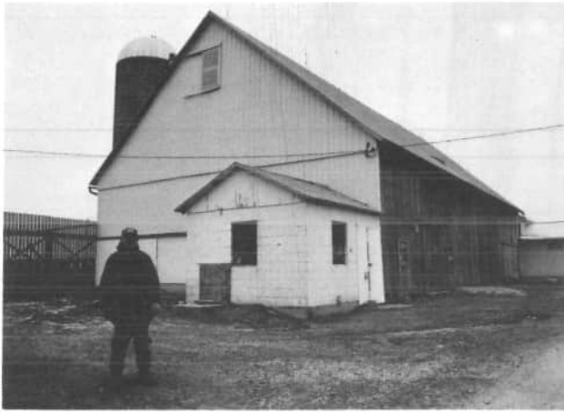
Bernard J. Franzer, standing outside his barn, at 5316 Carthagena Road, in January 1991. Today, the barn houses cattle, and stores hay and straw; there are large stables which can be cleaned mechanically.
