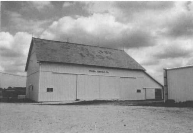
Russell Ferguson is written on the front of the barn, above the double doors, which identifies today's owners Russell and Ruth Ferguson, 9442 Erastus Durbin Road, Rockford. On the roof is written G. B. Jr., 1896, which identifies the owner George Bollenbacher who built the barn in 1896.
