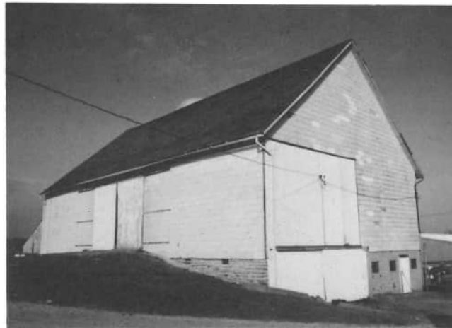
Urban and Mildred Knapke's barn, 2165 Rolfes Road, Maria Stein, was built in 1894 by Henry Menker, who was known for barn building. One can see the stone foundation, next to the bank leading to the double doors. It appears as if the main cross beams are extending beneath the eaves, above the double doors. This barn has been used for cattle, and hay storage.
