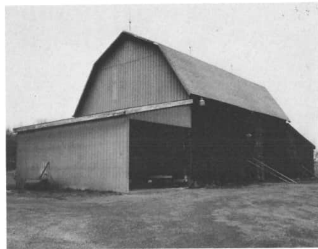
Jerry and Catherine Rasawehr, 11585 Elgin Road, Mendon own this barn. The barn was built before 1929. A family named Rexroat lived here, but it is not known if he built the barn. The barn has been used for animals, hay and straw and machinery. Today, it is used for machinery storage. The red barn, with its gambrel roof topped with three lightning rods, has a shed built to each end.
