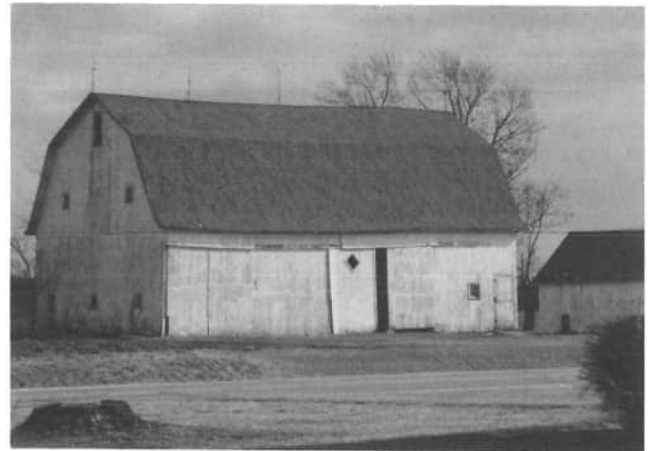
John and Cheryl Opperman's barn 9554 U.S. 127 North, Celina, was built in the 1800's. Five lightning rods are across the green gambrel roof. A larger window is at the peak of the end wall, while smaller, square windows are across the level of the mow, and across the ground level. One tipped window is still in the one sliding door. This sliding door has a slight overhang above it, protecting the door and the track from the weather. (Dave Slusser Photograph)
