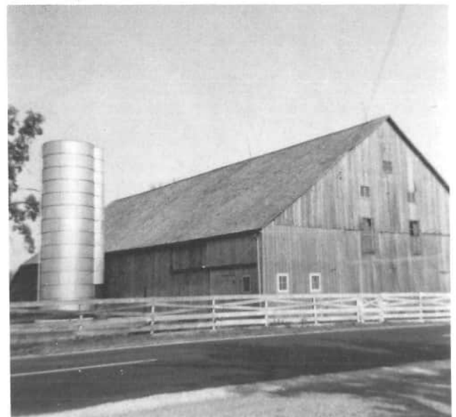
Ben Uhlenhake and carpenters built this barn at Donald Unrast's farm, in the early 1900's. The barn was used for livestock. This photograph shows the barn before anything was done to it. Notice the configuration of the three small windows in the gable end.
