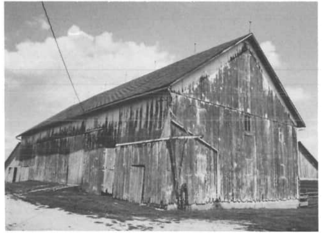
This barn was built a year before our nation's centennial, in 1875 by a Mr. Colus. Seven lightning rods, with their glass globes intact, stand tall across the ridge of the gable roof. Louvered vents are spaced along the top of the front wall. This barn, forty feet wide by ninety feet long, has oak frame work, with hand hewn beams, pinned with wooden pins. The barn has a wood floor in about three quarters of the barn and has two drive ways. This barn has been used for cattle, horses, and storage for straw, hay, and machinery. Today, the owner, Edson Pierstorff, 3701 Frahm Pike, Celina, uses the barn for grain and machinery storage.
