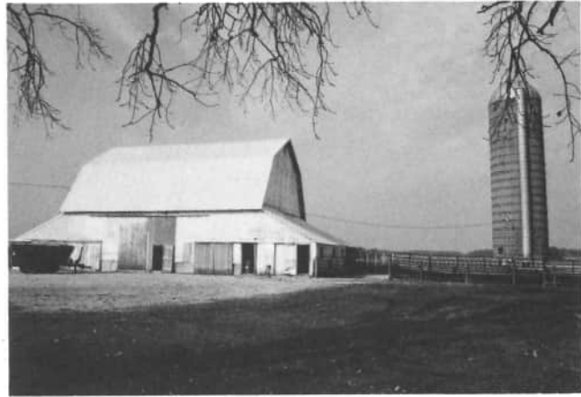
Glenn Heyne's barn stands at 4201 Monroe Road, Celina. This gambrel roofed barn has additions at both ends. The main double sliding door, has a smaller door, within this door; this smaller door is known as "le petit guichet."
