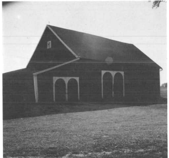
The afternoon sunlight, in the springtime, is casting a slight shadow across the front of the Charles M. Putman barn, 3009 State Route 29, Celina. This gable-roofed barn is painted red, with white trim and white arches on the two sets of double doors. This style barn is sometimes called an English barn, with a shed added to the left side. In the past, the barn was used for raising livestock; today the barn is used for storage.
