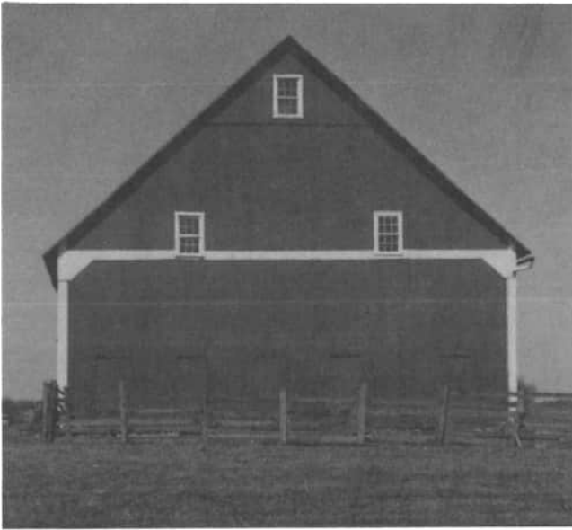
An end view of Eleanora Moeder's barn, which shows the five stable doors. Three windows are placed in the triangular configuration in the gable end, for light to the interior. The corners and roofline are outlined in white. (Auggie Jutte's photograph, which states "Grandpa Joseph Moeder's barn" on the back of the photograph.)
