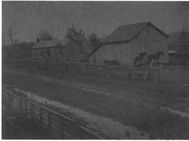
This barn may have been the Riley Homestead on what is now State Route 703 and Riley Road intersection.
