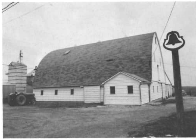
Ray Stachler and Bernard Siefring, Sr., with the help of the Siefring Brothers, built this barn, using lumber from their farms in 1954. The barn was built quickly because of the nice weather. In the past, the barn was used for milking and hay and straw storage. The barn is being used for storage and hogs by today's owner, Bernard Siefring, 5130 Burkettsville St. Henry Road, Coldwater. The barn stands on the east side of the road. The dinnerbell in the foreground has called many farmers to the dinner table.
