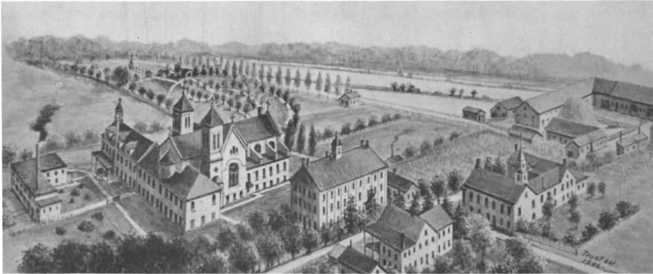
Drawing by Father Paulinus Trost in 1906 laundry, convent and chapel, Old Seminary , Brothers' House, Old Abbey , barns (The present main building is to the right of the chapel and the Old Seminary )
