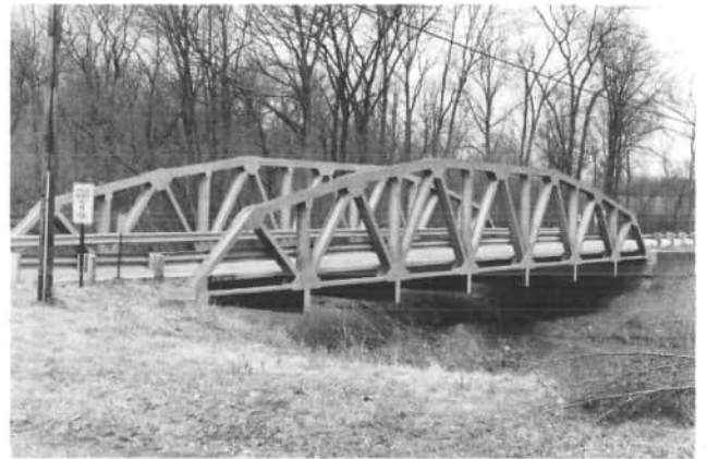
The Celina Mendon Road Bridge over Twelve Mile Creek is a Sloping Top Chord Warren Truss built in 1955 by the Ohio Bridge Co. of Cambridge, Ohio. This early example of a modern style is still an occasional new bridge design at the local level.
