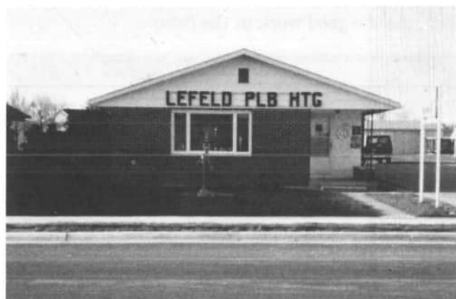
Lefeld Plumbing & Heating
