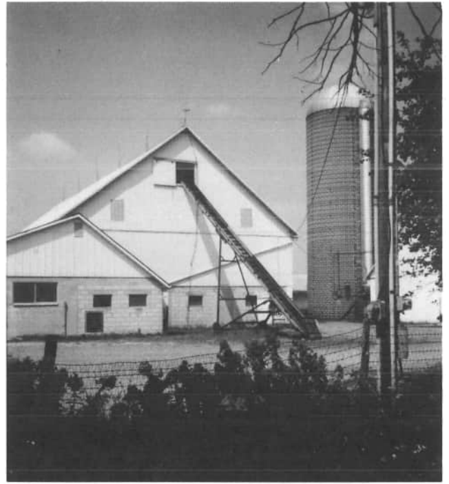
Henry Feldhake and hands built this barn, in 1902. The barn was used to house their work horses, a few cows, and loose hay and grain. Today, the barn is owned by Clarence and Shirley Heuing, 3389 Fort Recovery-Minster Road, Saint Henry. The barn is used for dairy cows, and baled hay and straw. In the photographs, the elevator is placed to send the bales up to the mow, through the door, which slides on the tract to the left. Six lightning rods grace the ridgeboard of the gable roof.
