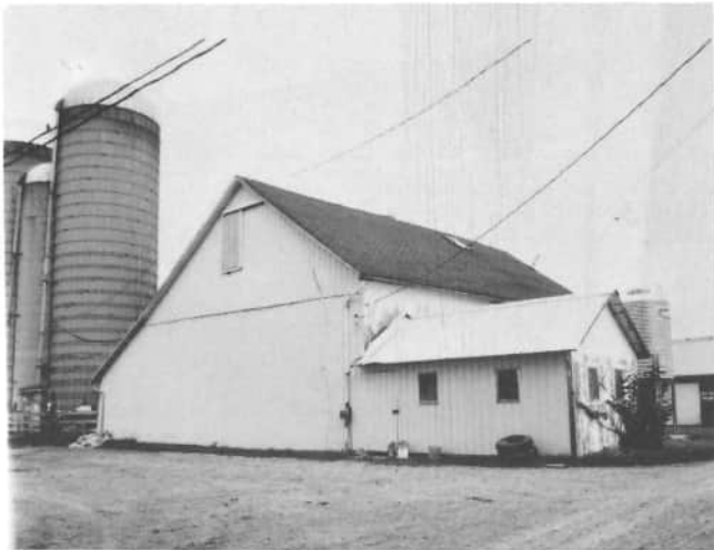
Robert Guggenbiller's barn, 2577 Fox Road, Fort Recovery, was probably built before the Civil War, sometime in the 1850's or 1860's. The barn is 65 by 43 foot. Today, the barn has free stalls with hay and straw overhead. (Andrew Pax photograph)
