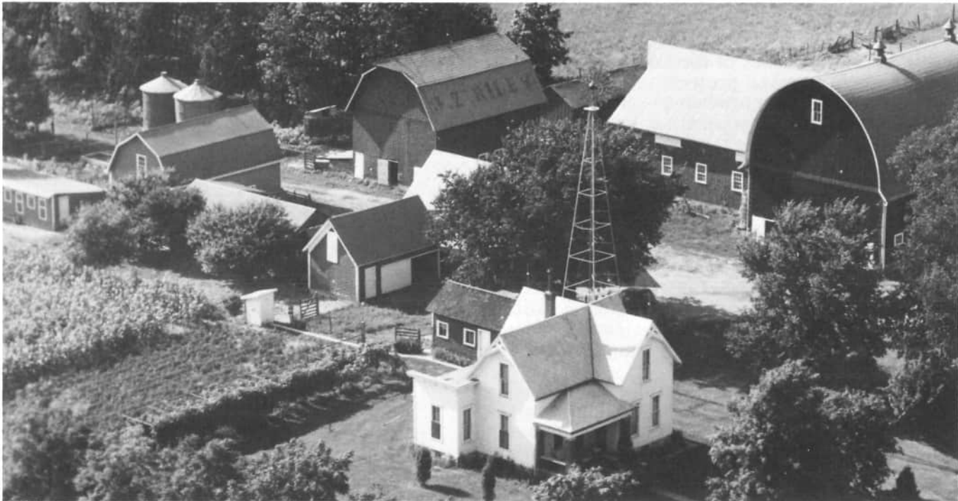
C.E. Riley or J.Z. Riley built this barn at 7239 Riley Road, Celina, in the early 1900's. The main barn has the round roof, with two ventilators on top, and has an addition to the back, with a gable roof and triangular hay hood. This barn was used for dairy and hay storage. The smaller barn in back of it, has J Z RILEY in the slate of the gambrel roof. The windpump (windmill) can be seen standing next to the house. The home and the other out buildings complete the rural landscape. Today the place belongs to David Riley.
