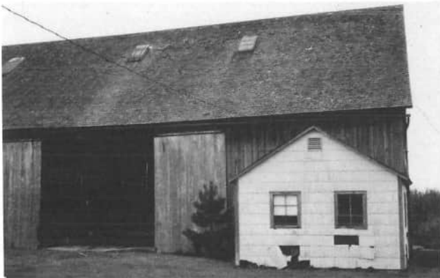
This is the appearance of the barn at 3277 Goettemoeller Road, Celina, when Jerry Will Jr. purchased his farm from Gregory Schaefer in September of 1986. The barn had its original shingle roof and siding. Since Jerry bought the farm, he has been slowly remodeling the barn by replacing the roof, siding, and removing the old milking parlor, and remodeling the interior for swine production.
