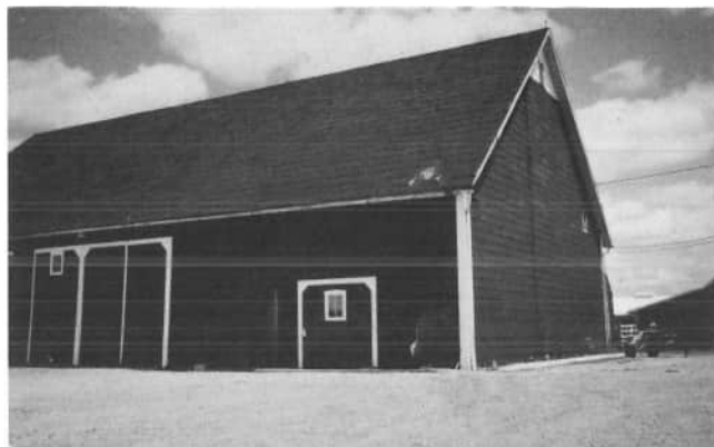
Donald and Edna Kremer, 8549 St. Rt. 274, New Bremen, own this barn in Marion Township. This red barn, with the white trim on the doors, corners and gable end, was built in 1909 by a man named Menker. Both the large and small sliding doors have windows for interior lighting. The barn was originally used to house milk cows, hogs, and to store hay, straw and grain. Today, the barn is used for cattle, hogs, and to store hay, straw and grain.
