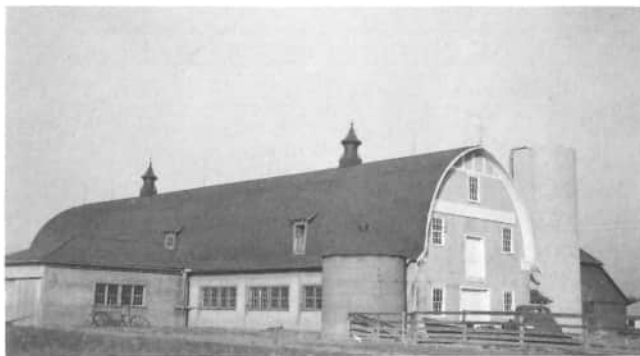
The "North Shore Stock Farm" of Dr. Robert E. Riley, 2015 State Route 703 East, was noted for registered Holstein and Guernsey Cattle. This barn was the centerpiece of the farm. The barn had stanchions for dairy cattle, as well as the large area for hay storage. (photograph from Joel K. Riley)
