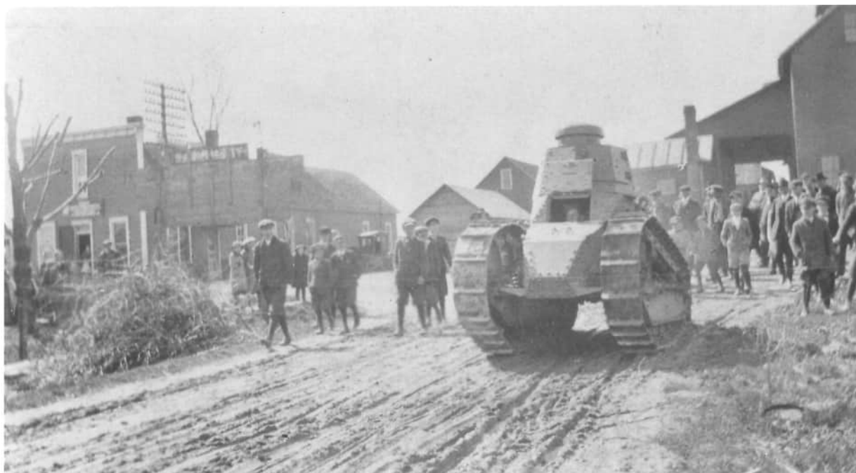
1917 - Back left, the Maria Stein Lumber Co.; back right, Maria Stein Grain Co. (8010 St. Rt. 119).
