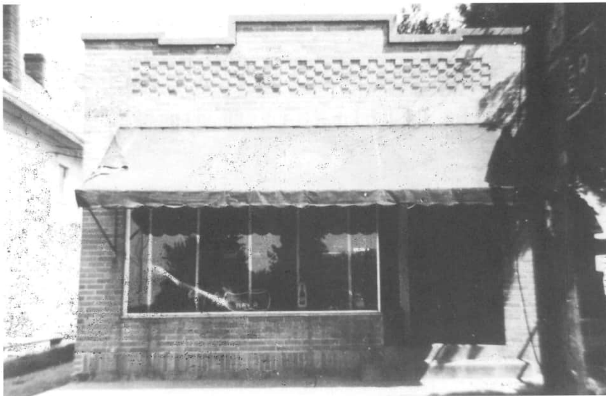
About 1945 - When Joseph Gast sold the beer stube to the Knights of St. John in 1941, he built a new beer stube between the house and the Knights building. When this building was dismantled, it became part of the Louis Overman dwelling.
