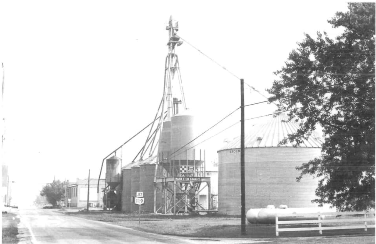
1978 - Maria Stein Grain Co. from about the same position as the above photograph.
