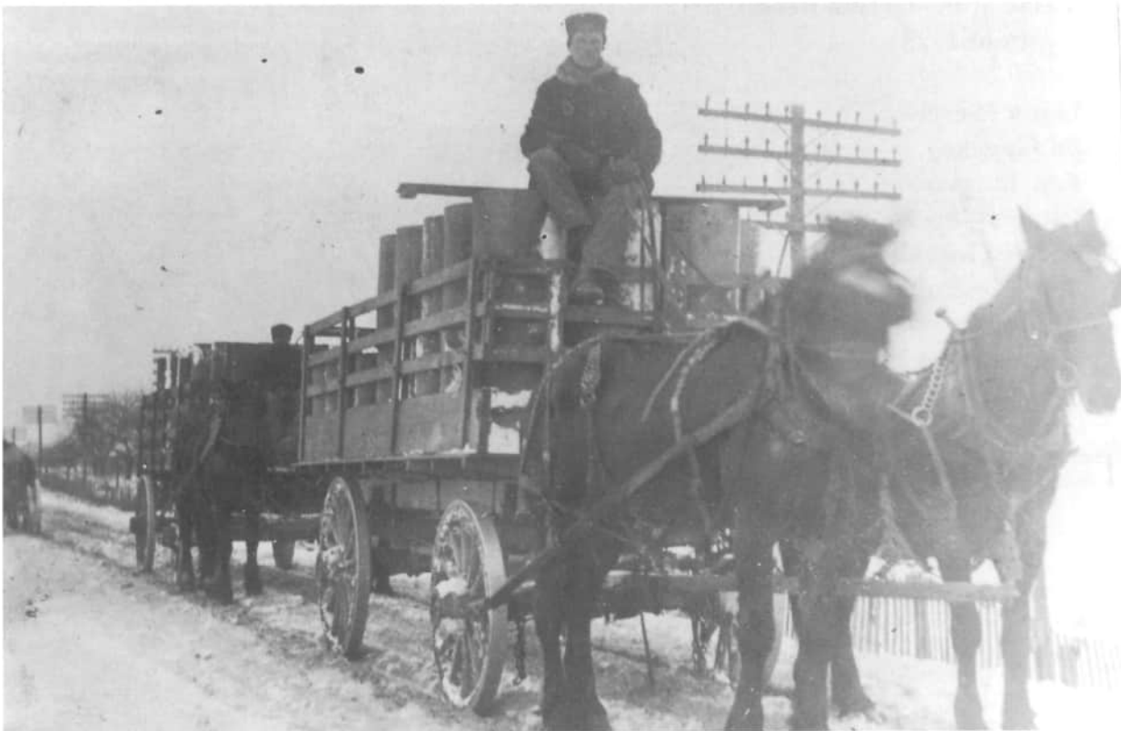
About 1916 - Ben Tangeman, Sr., hauling tile for the Goecke Tile Yard.
