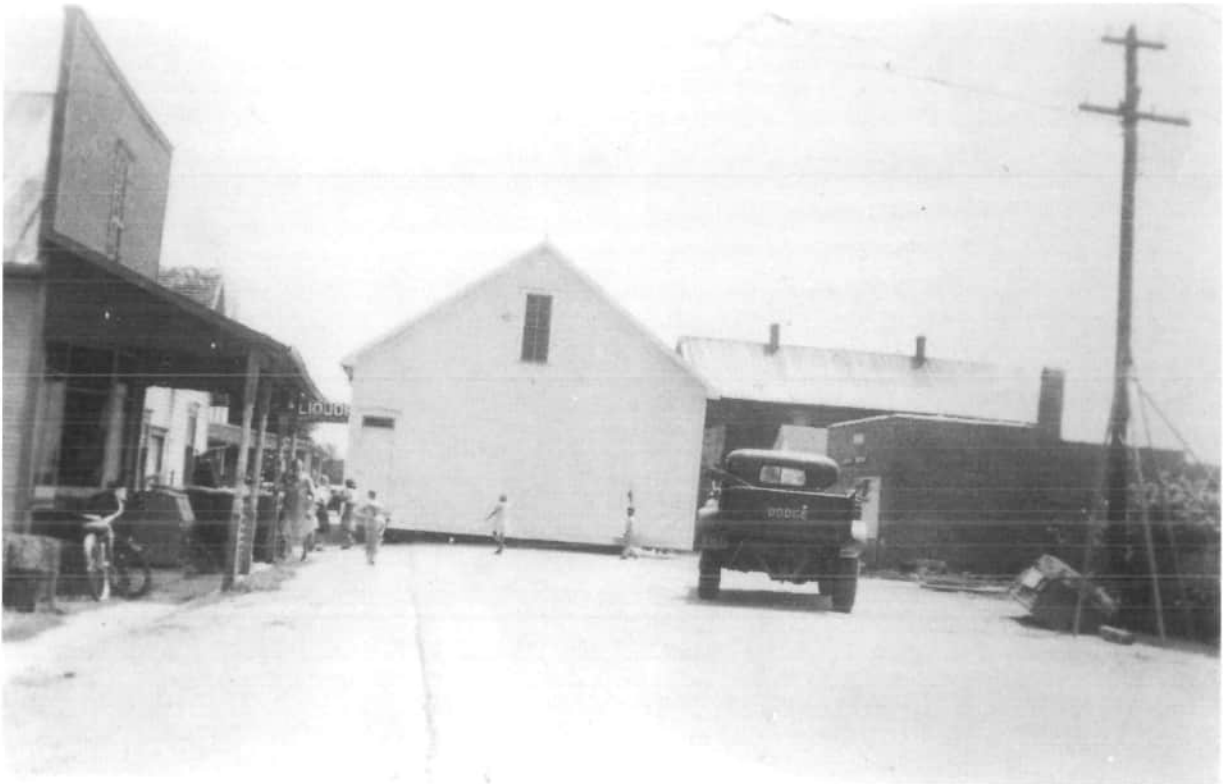
1949 - The Community Hall being moved down the highway a fourth of a mile to its new location on the Legion grounds (8140 St. Rt. 119).
