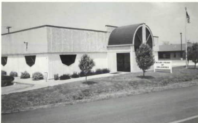
Miami Tribal Office Building and Senior Citizen Center Miami, Oklahoma
