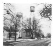
Construction of the new water tower for Saint nry was completed in the autumn of 1971. The v water tower was 140 feet tall and held 150,000 lons of water. The rust removal plant was comted in 1973 at a cost of \$70,000.
