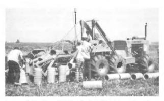
Picture of a Speicher 7060 Trencher installing a concrete main on the Dull Farm in 1978
