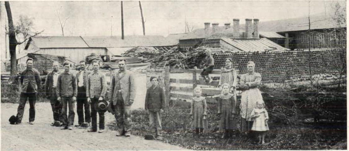
A RECENT VIEW OF THE PLANT
