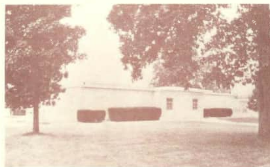
Mersman Swimming Pool building
