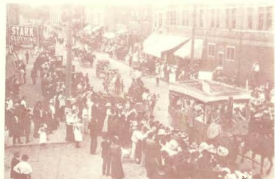
View of West Fayette Street.
