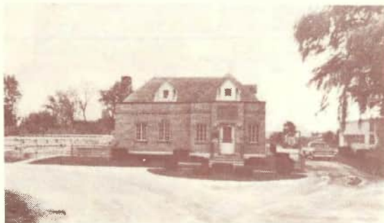
The Celina Sewage Treatment Plant, designed to handle a flow of 900,000 gallons per day of domestic and industrial wastes, went into operation on February 15, 1940. In 1962, it was expanded to a capacity of 2,000,000 gallons per day.
