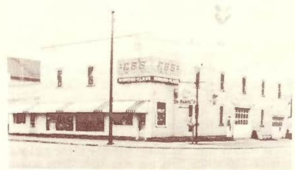
C.B.S. Automotive Supply Inc., 401 South Main, was begun in 1949, by A.J. Schritz, Otto Steinbrunner, and Dale Baer. (J. Wenning, early saloon site) (See photos — 1930's)
