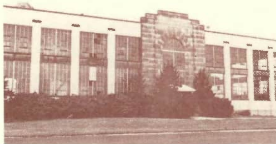
The Celina Municipal Power Plant was constructed in 1941; the old plant on Touvelle Street was retained on a stand-by basis.
