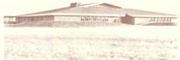
The Cheryl Ann School, Mercer County Mental Retardation Program, was built in 1976 on the corner of Fleetfoot Road and Mud Pike. Fanning/Howey & Associates were the architects.
