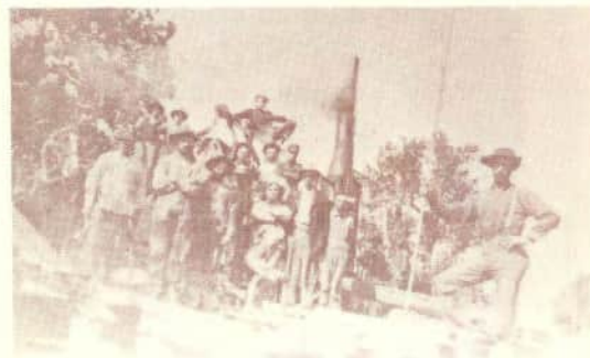
Building the West Bank on the Reservoir.
