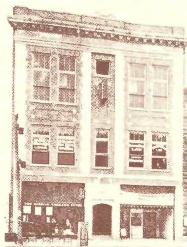
Odd Fellows Building, located East of First National Bank, on West Market.
