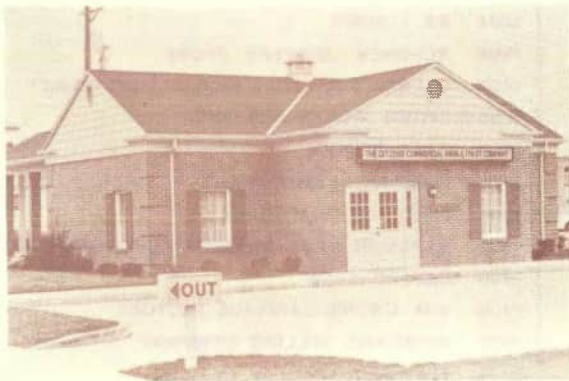
Citizens Commercial Bank and Trust Co., Fayette Street Branch Bank, opened August 1981.
